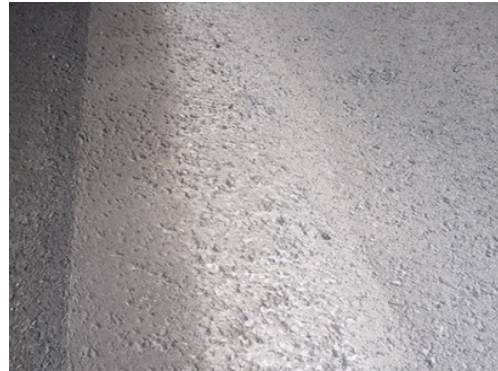
Figure 4.2: Poor Eradication of Temporary Pavement Markings
