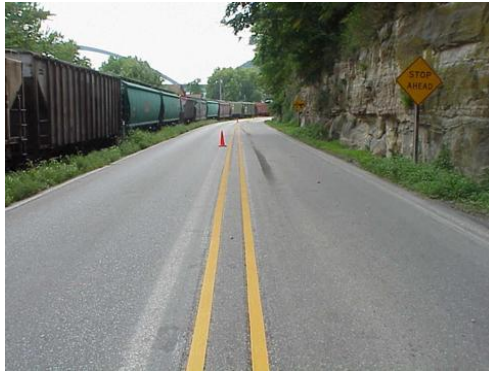
Figure 4.2: Poor Eradication of Temporary Pavement Markings
