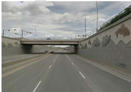
Example of a trenched road with a local connection overhead. Local traffic, pedestrians and cyclists can cross the highway without changing elevation.
