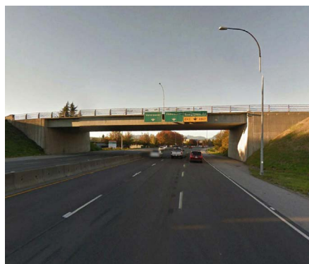
Example of a grade separated crossing (overpass) over a highway. This provides a local connection for all modes without access to the highway.
