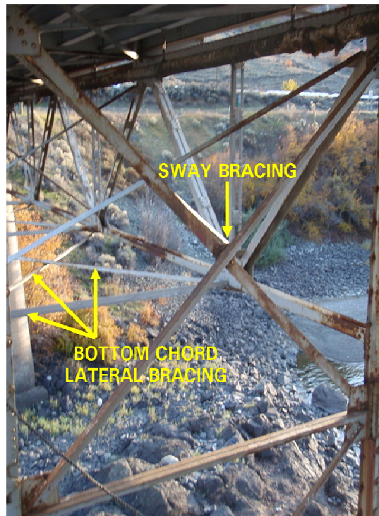
Figure 4: View of Typical Truss Span Showing Lateral Load Carrying Members
