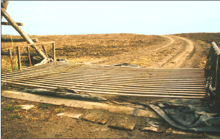
Figure 12 Spring-Supported Temporary Cattle Guards
