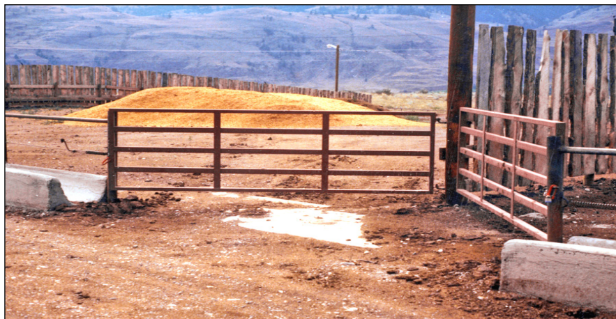
Farm-Built Woven Wire Gate
