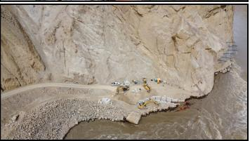
**TOP:** Installation of anchors that will suspend the tubes for the pneumatic fish transport system
