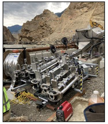
**PICTURED:** Installation has started on Phase 2 of the Whooshh Passage Portal<sup>™</sup>. Top right: the scanner box component assesses each fish entering the pump. Centre: the accelerator directs the fish into the assigned tube.
