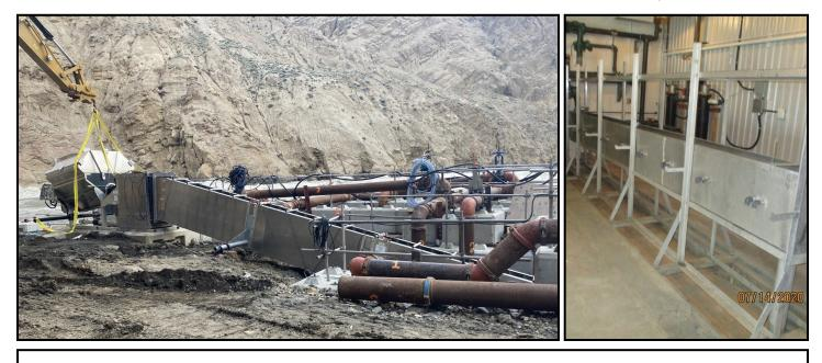
LEFT: Reinstallation of the Whooshh Passage Portal<sup>™</sup> components after water levels receded, including the steep pass and scanner skid.
