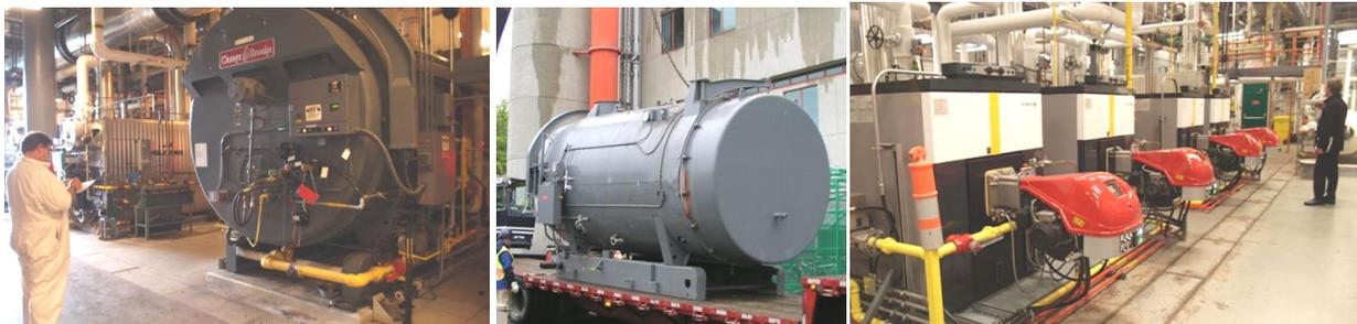
*Victoria General Hospital's two old boilers were removed and replaced with four high efficiency boilers*
