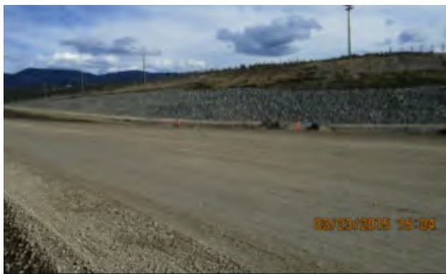
Rip Rap Slope Stabilization Treatment
