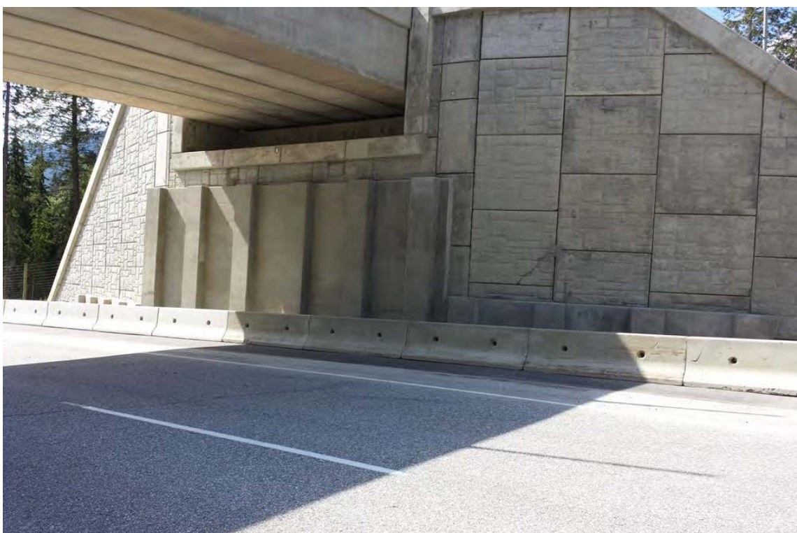
MSE Wall Repair Complete 2014
