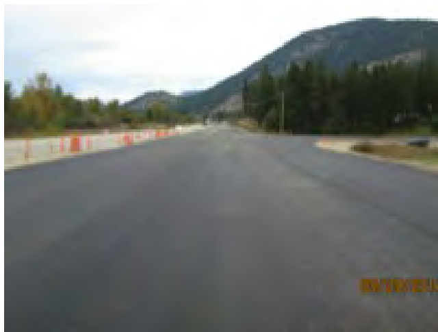
Bottom lift paving of L100 EB lanes
