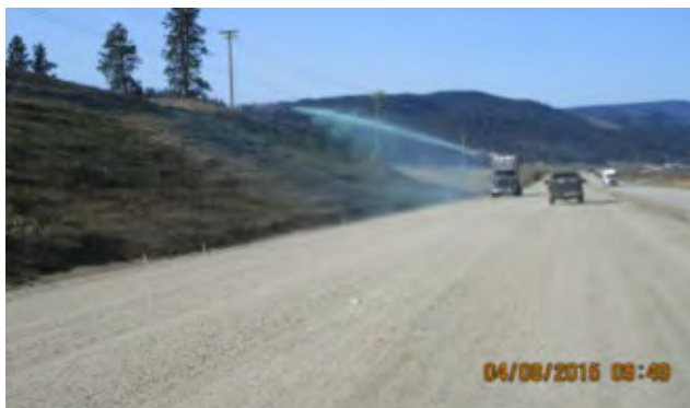
Hydro Seed Slope Stabilization Treatment
