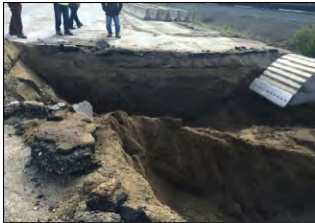
Double Layer of Lift Asphalt in Existing Four-Laning
