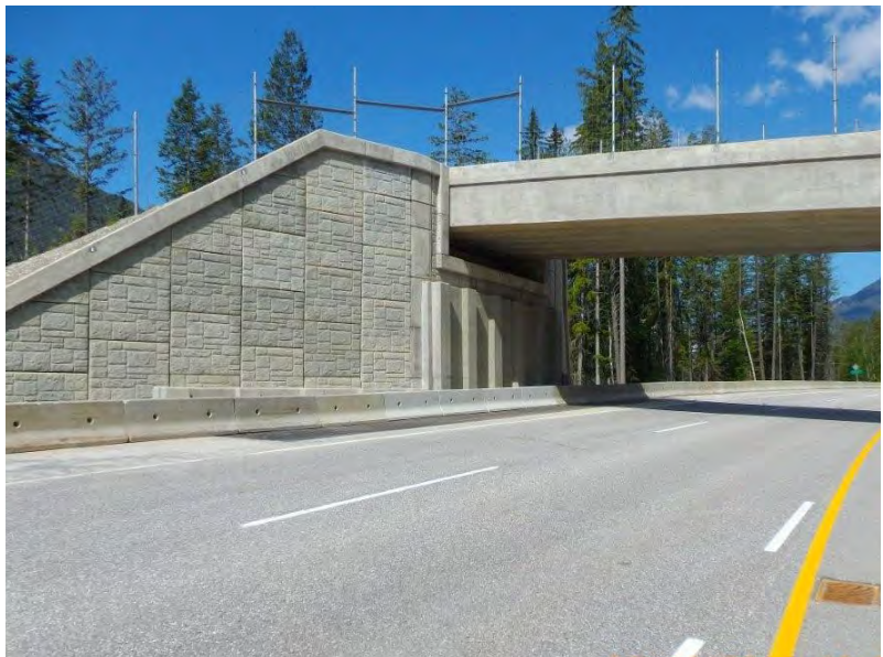
MSE Wall Repair Complete – Glenogle 19 June 2014
