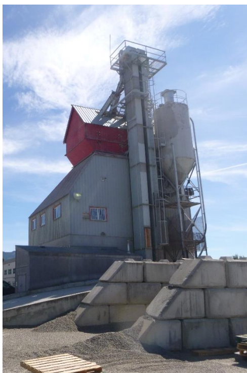
Photo of silo with air pollution control works on top (baghouse filter)
