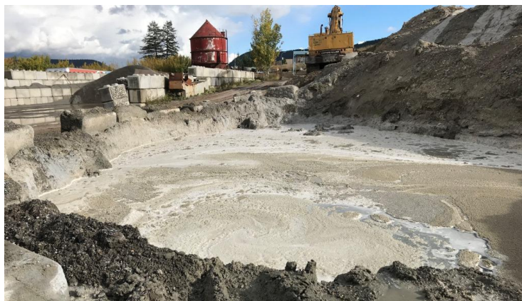
Photo of infiltration pond at concrete facility
