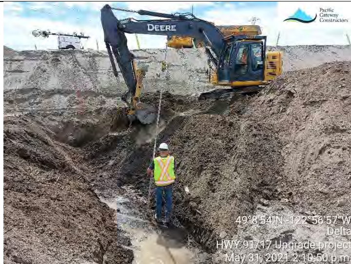
Photo 11. L575 (E). Placing STM 225 & 330.
