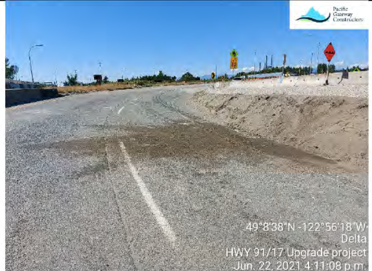
Photo 2: Asphalt staining residue remained after completion of the spill-cleanup
