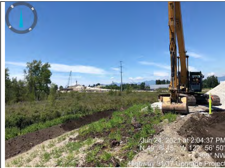
Photo 23. L1170 (F). Peat berm placement completed.
