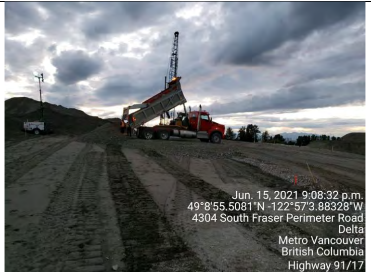
Photo 12. L575 (E). Placing final grade gravel.
