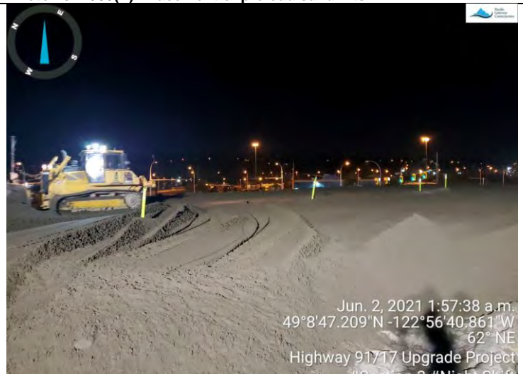
Photo 20. L500 (F). Greenbelt placing sand.
