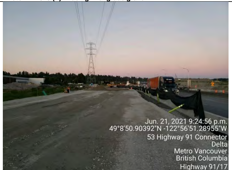
Photo 14. L575/500 (E). Gravel placement and dust suppression.
