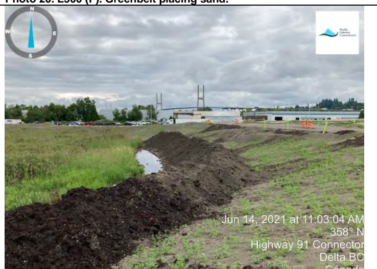
Photo 22. L1170 (F). Peat berm added to the bottom of sand slope.
