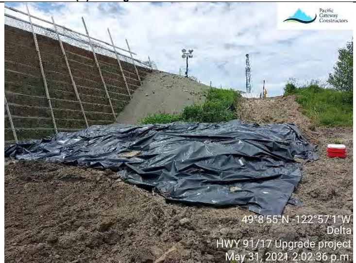
Photo 10. L575 (E). Suspect contaminated soil covered in poly.
