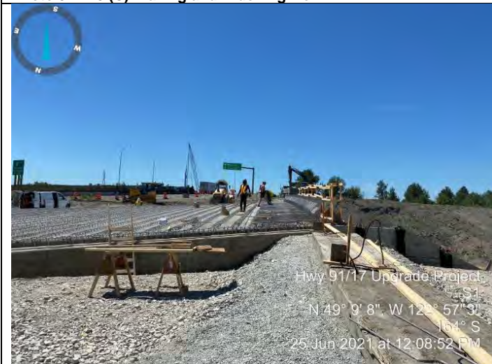
Photo 7. S1 Bridge (C). Rebar installation.
