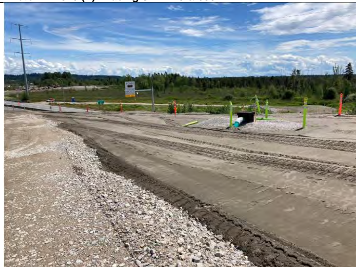
Photo 13. L500 (E). Installed catchbasin.
