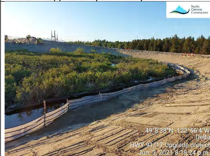
Photo 25. L2400 (G). Inspection of ESC fences.
