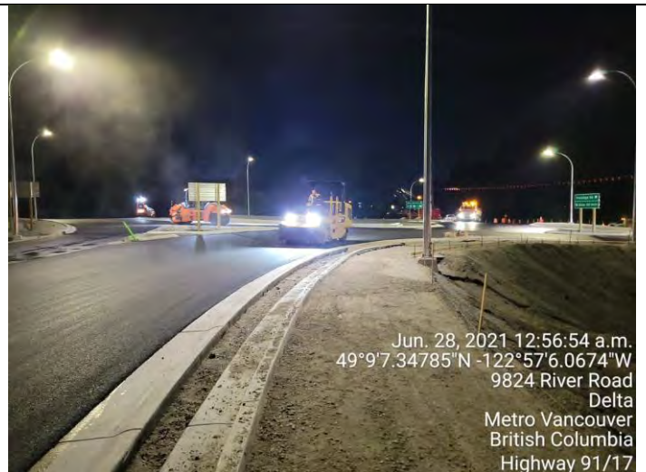
Photo 8. L250 (C). Paving the roundabout.
