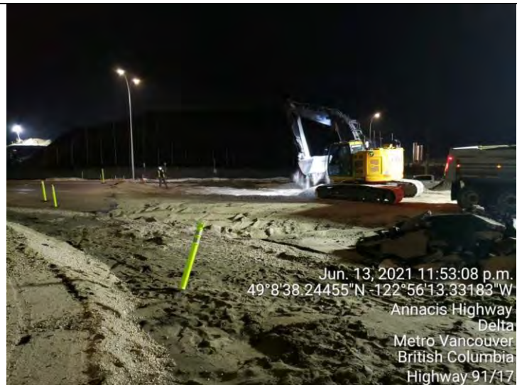
Photo 26. L600 (I). Placement of preload sand.
