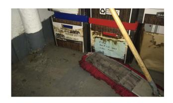
During a heavy rain event, the water table rose above some underground conduits that connected services. As the conduits were not water tight and the basement is lower the conduit directed water into the basement.
