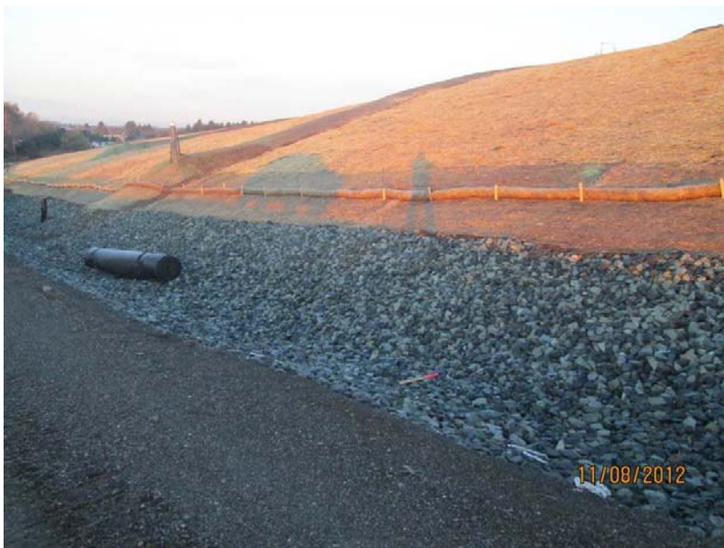
Photo 6-2 Erosion Control Measures on Phase 2 at Vancouver Landfill
