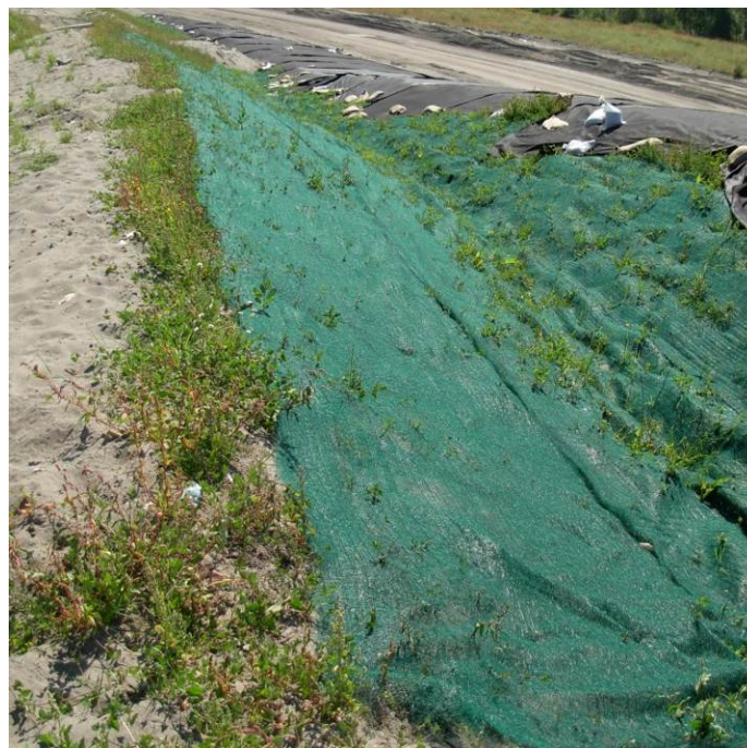
Photo 10-5 Erosion Control Blanket in a ditch at the DSS Landfill in Delta.
