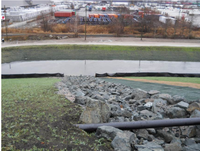
Photo 8-2: Delta Shake and Shingle Landfill Downchute
