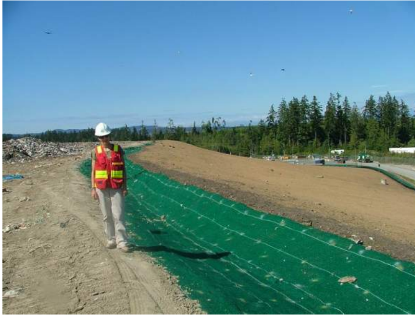
Photo 8-1: Erosion control matting in use at Nanaimo Landfill
