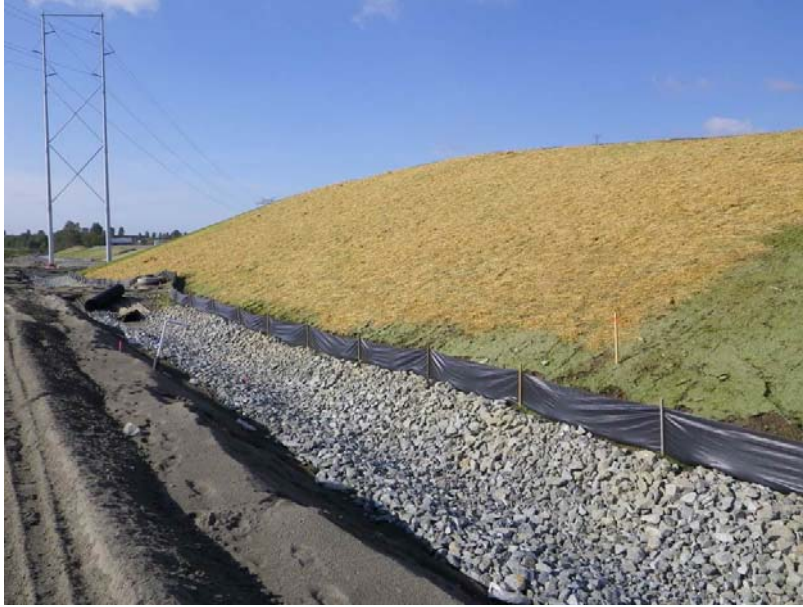
Photo 10-3: Loose Straw Application on DSS Landfill in Delta.
