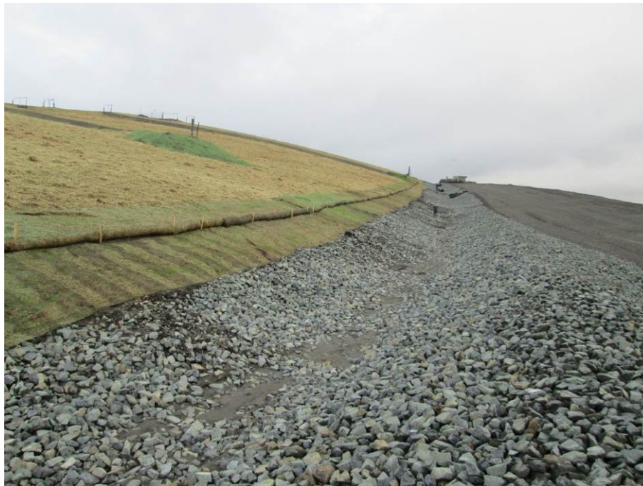
Photo 10-4 Erosion control on slope and ditches at the Vancouver Landfill
