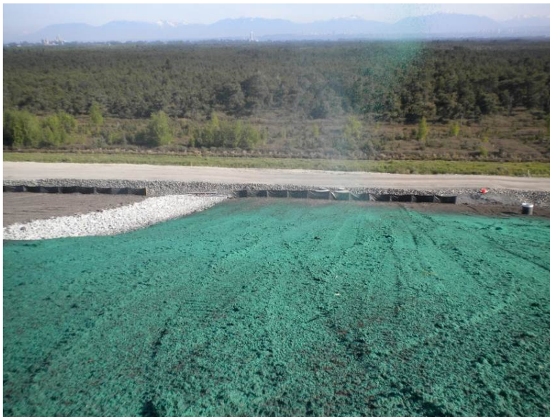
Photo 10-1: Vancouver Landfill Phase 1 Hydraulic Seeding Application
