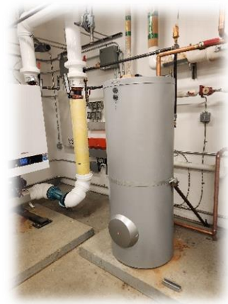
Figure 4 – New Queneesh indirect water heater
