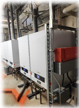
Figure 1 – New condensing boilers at NIDES
