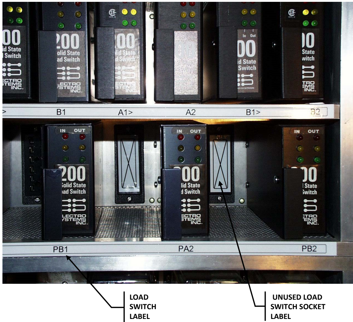
Figure 9. TS1 Typical Load Switch and Unused Load Switch Socket Label
