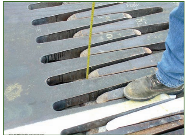
New Ten Mile Bridge Expansion Joint
