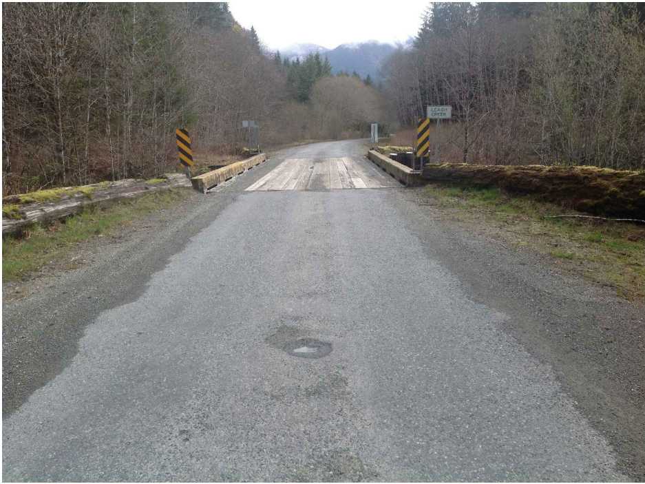
APPROACH FROM WOODS (LEFT) SHOWING CHIP SEALED RUNNING SURFACE
