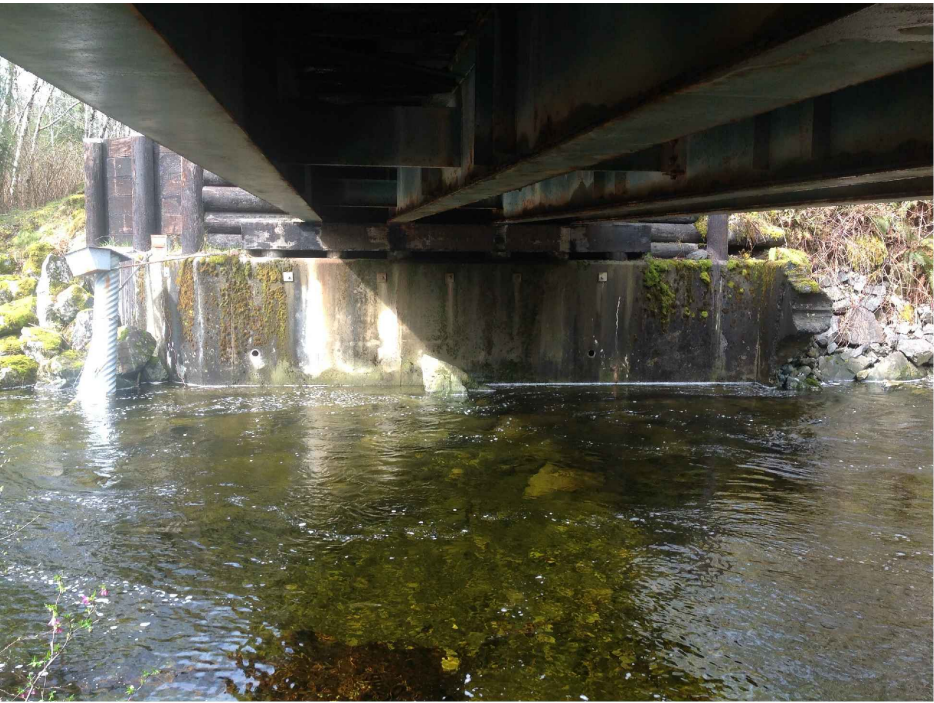
TOWN (RIGHT) ABUTMENT SHOWING EXISTING CONCRETE TO BE REMOVED
