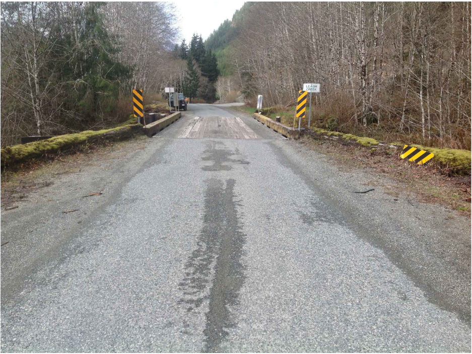
APPROACH FROM TOWN (RIGHT) SHOWING CHIP SEALED RUNNING SURFACE
