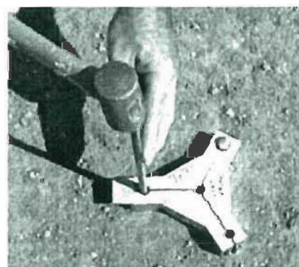
FIG. 5 Driving Spikes Through Template
