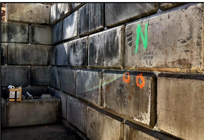
With the onset of the spring freshet, work is focused on the concrete fish ladder at the West Beach area of the site. Originally built last year, the structure is undergoing some significant upgrades. This past week crews completed the final placement of blocks to expand the ladder. They sealed and backfilled the blocks and poured the concrete base in the sedimentation basin. Handrails, wooden platforms and steel walkways are now being installed.
