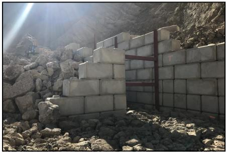
**TOP:** Preparations to install the tubes for the pneumatic fish pump system. **BOTTOM:** Concrete fish ladder construction is well underway, with over 500 blocks to be used in the final construction.
