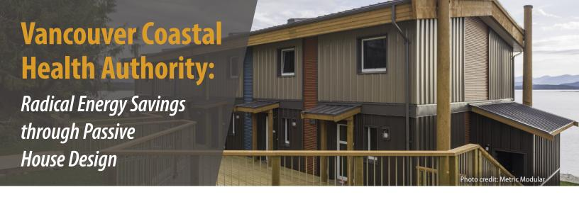
When a fire damaged the staff housing complex for R.W. Large Memorial Hospital in Bella Bella, the Vancouver Coastal Health Authority rebuilt the complex to Passive House standard as a way to significantly—and permanently—reduce greenhouse gas (GHG) emissions and energy costs. The project demonstrates that high quality, energy efficient buildings can be achieved in remote communities, reducing energy costs and reliance on GHG-intensive fuels.
