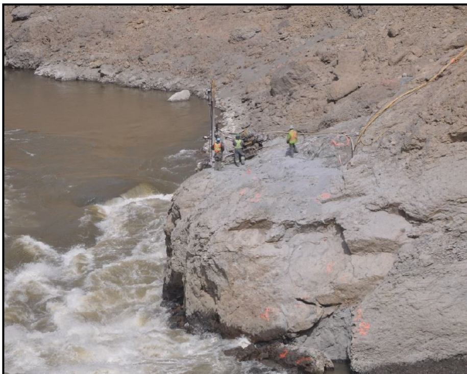
TOP: Aerial view of the site, including (L-R) the concrete block fish ladder construction, the completed “nature-like” fishway and the protective rock fall canopy BOTTOM: Crews drilling the East Toe in preparation for the second large blast, which will occur in April
