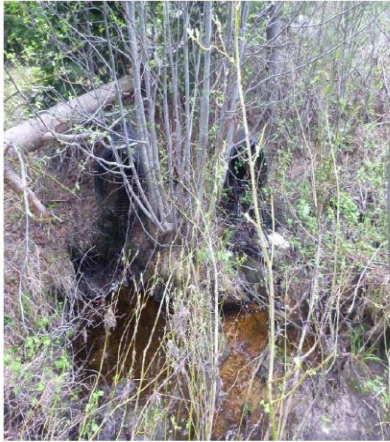
Photograph 1. View of two culverts downstream of the crossing location with limited flow due to blockage. (May 23 , 2018).
