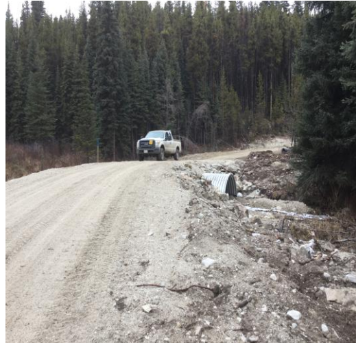
Photograph 1. View of two culverts downstream of the crossing location with limited flow due to blockage. (May 23 , 2018).
