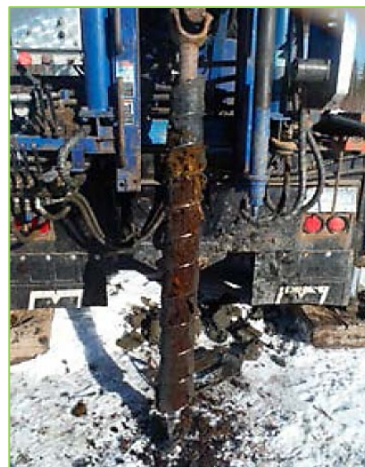
Figure 2 - Drilling in Support of Site Investigation (OGC, 2015)
