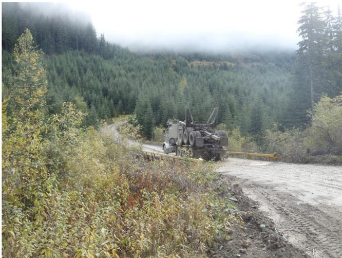
Figure 12. Middle Memekay Bridge, Branch C1000, site #320. Grader berms at this location concentrate road surface drainage onto the bridge where it flows directly into the Middle Memekay River.
