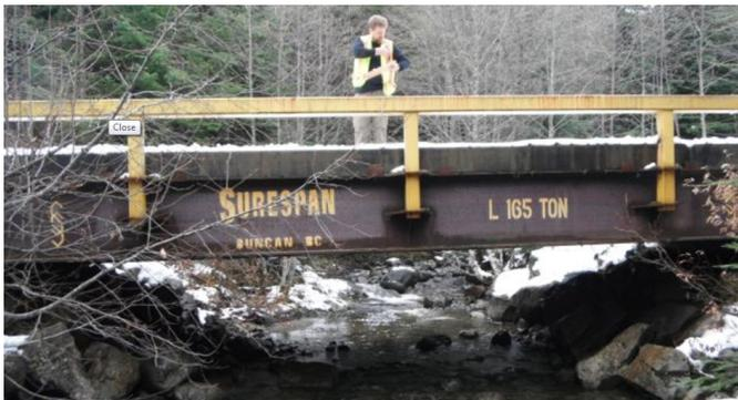
**Figure 8.** Located in the North Memekay, this small bridge (Crossing ID# 102823) crosses a 3rd order stream that has over 3km of upstream observed and modeled habitat, and is a good example of a crossing that easily passes fish, storm flows and debris.
