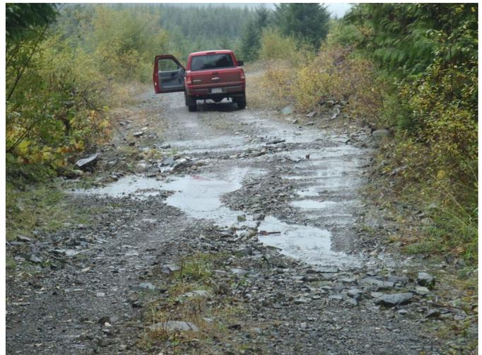
Figure 13. Cooper Main. On some inactive roads, relief ditches capture small streams, directing concentrated storm flows onto otherwise dry hillslopes. These have the potential to form streams with chronic sediment problems.
