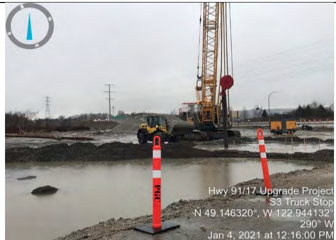
Photo 14. Stone column installation continued. Sand berm separates work area (shallow rainwater) from deep pool of water between sand alignments at the L1150/L500 (F).
