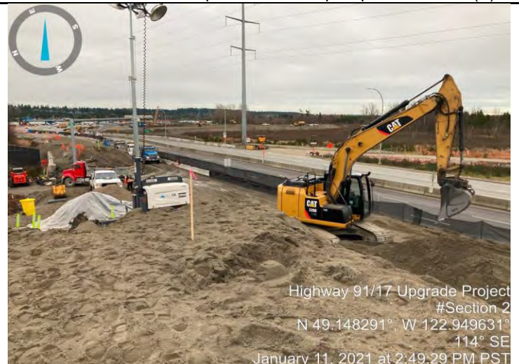
Photo 12. Importing and placing sand and lock blocks at Wall 210 (E).
