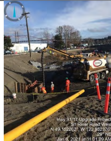
Photo 2. Separate area of Fortis gas line excavation. Yellow pipe being fused for tie-in at River Road West (C).
