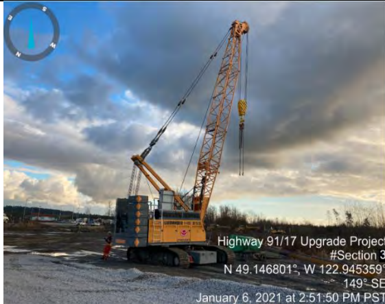
Photo 15. Menard assembling new crane for further stone column installation at the L1450 (F).
