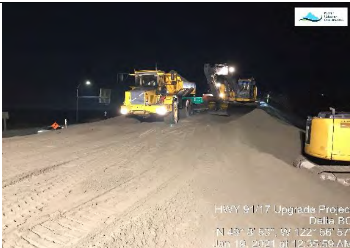
Photo 13. Preload placement and compaction continued at the L500/L575 (E).
