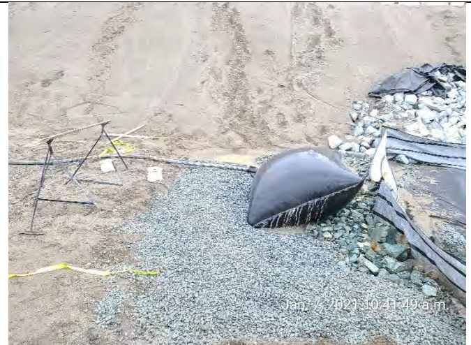
Photo 26. Filter bag at end of discharge hose - River Rd West (C).
