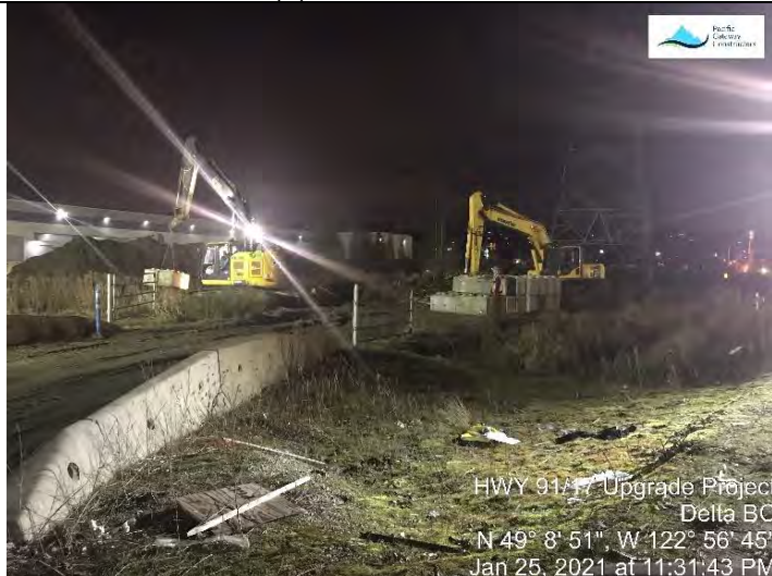
Photo 17. Placement of lock block wall commenced at the L1300 (H).
