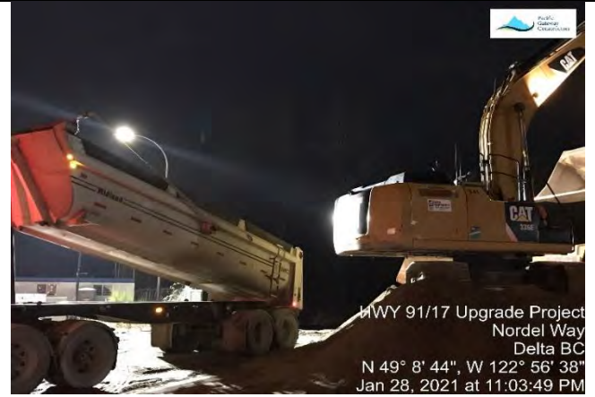
Photo 16. Stockpiling, relocation, & placement of preload sand at the L1150 (F).
