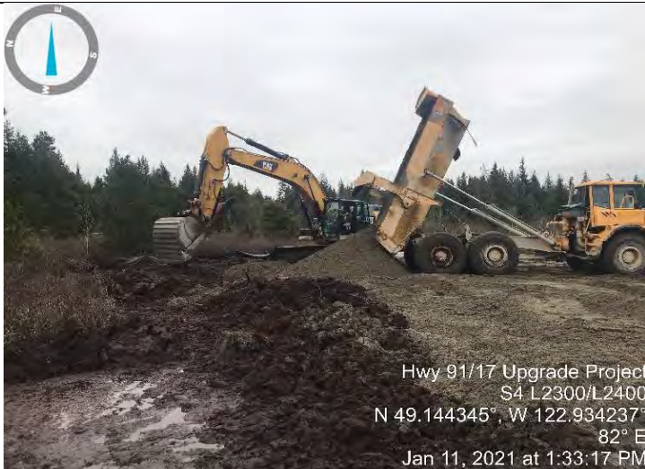
Photo 19. Clearing & padding out sand to build out alignment that extends over removed boardwalk area at the east end of L2300 (G).
