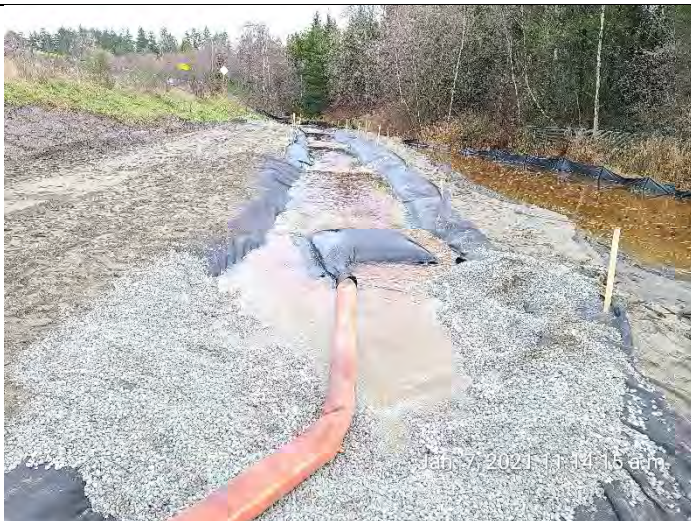
Photo 23. Pumping at north end of L2300/L2400 (DNR)(G). Flows from 6-inch pump dewatered through filter bag and into clear crush spillway.
