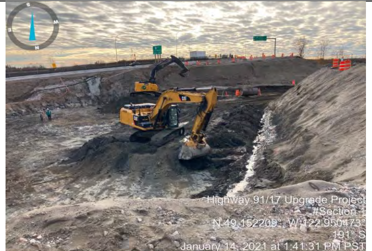
Photo 4. L500 – Walls 202 and 210 (E). Preload bordering Hwy 91C continuing to be built up and pulled out to the east.
