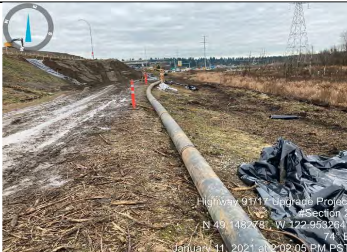
Photo 11. 200 mm culvert to be installed running along west side of Hwy 17 (E).
