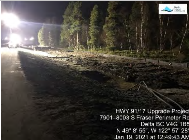
Photo 7. Preload placement and infilling of roadside ditches continued at the L100 (B).
