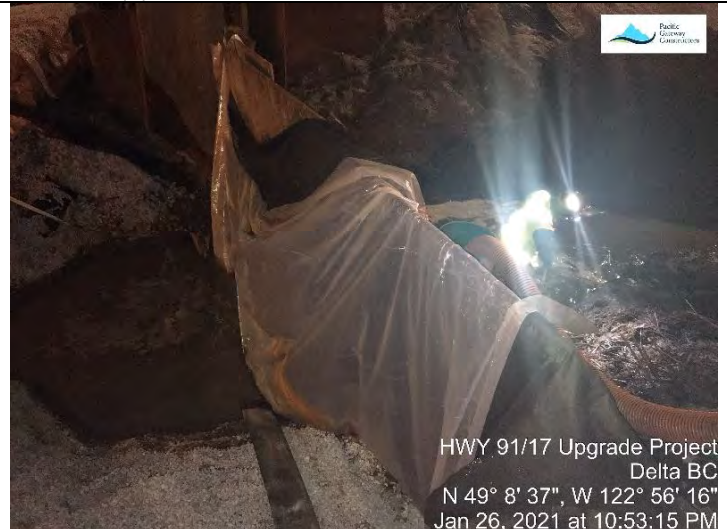
Photo 18. Dewatering into temporary cofferdam at the L2100 (I).
