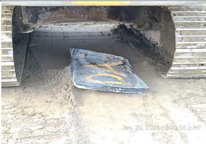
Photo 5. Some spill trays were damaged and were no longer functional.
