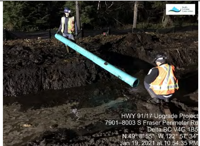
Photo 8 Installation of CB extensions at the L100 (B).
