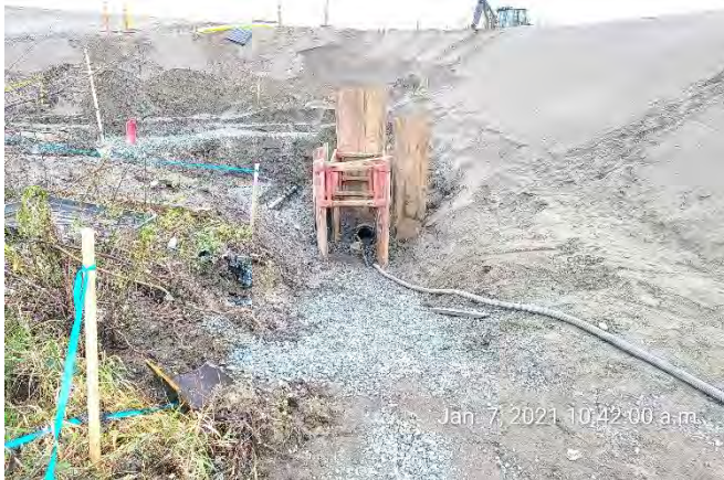
Photo 25. Clear crush sump in utility trench - River Road West (C).
