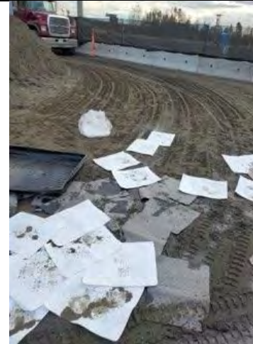
Photo 22. Spill pads applied immediately on ground at the L500 preload sand delivery area north of Hwy 91C (E).
