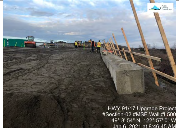
Photo 10. Lock block wall placement on top slope of Wall 210 (E).
