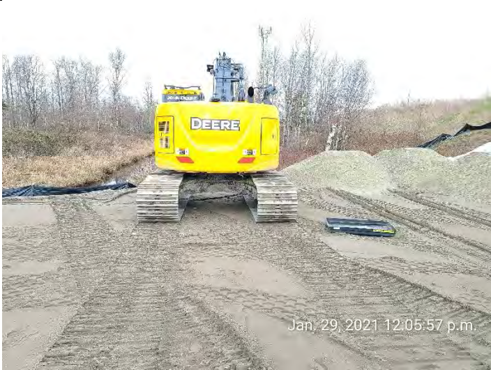
Photo 31. Spill trays were often lacking from idle equipment despite being readily available.
