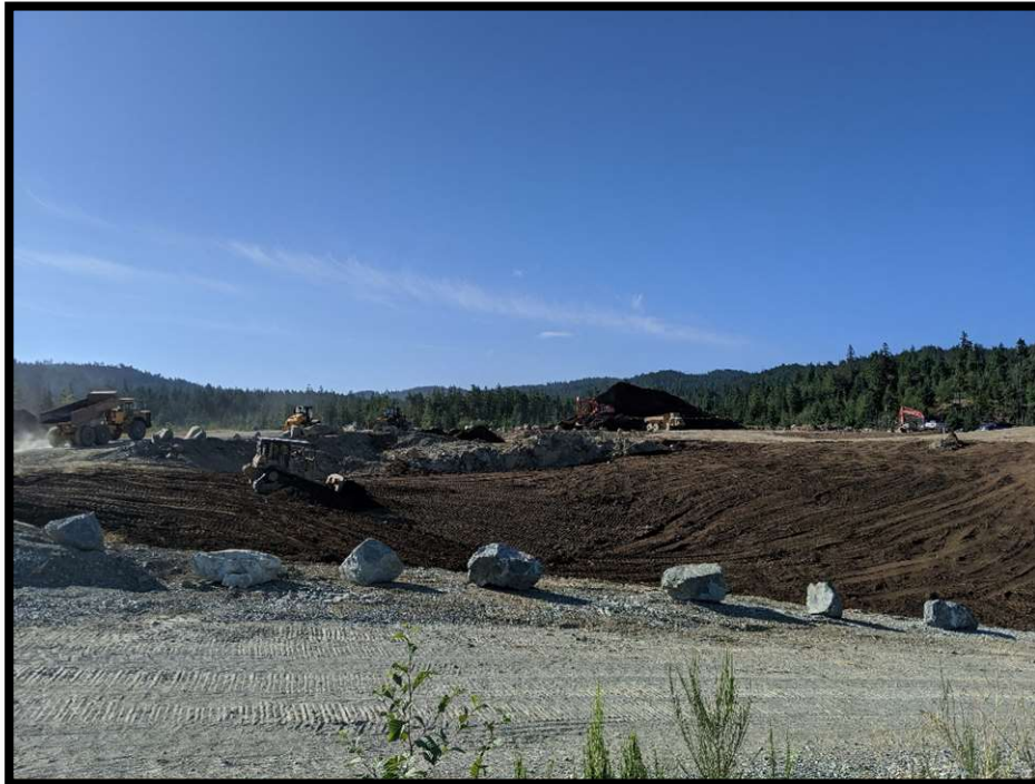
Picture # 1: Looking south towards topsoil material being graded out along the south side of the leachate facility access road. The final lift of PEA topsoil is expected to begin placement tomorrow and will be assisted by an on-site surveyor to provide spot elevations. Hydroseed placement is scheduled for Thursday August 27, 2020.
