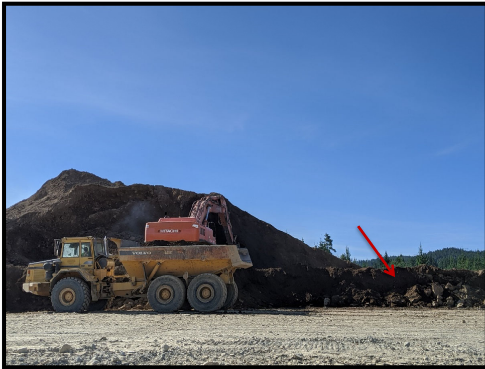
Picture # 3: Larger rocks were sorted out of the topsoil material (red arrow) prior to loading into the rock trucks for material transportation.
