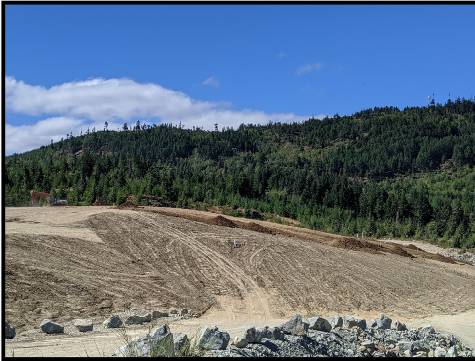
Picture # 1: Site overview looking southwest towards topsoil placement along the north and western sides of the PEA. Two rock trucks hauled material throughout the day to various locations to be graded out with an excavator, and bulldozer.
