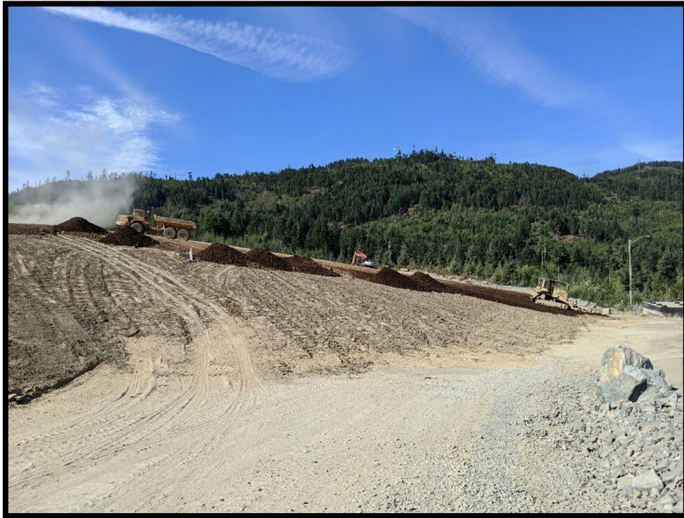
Picture # 1: Site overview looking southwest towards topsoil placement along the north and eastern sides of the PEA. Two rock trucks continued to haul material throughout the day to be graded out with a bulldozer.
