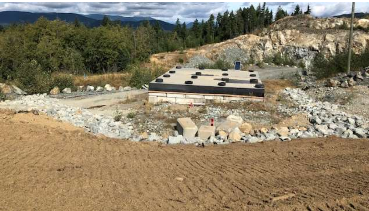
Picture #5: Toe ditches complete at north slope
