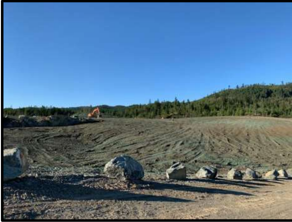
Picture # 1: Looking south towards hydroseeded PEA and rip rap that has been placed to delineate the edge of the road.
