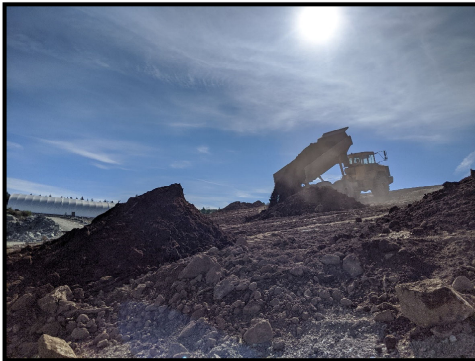
Picture # 4: Looking east along the north side of the PEA towards topsoil material being bulked in prior to being graded out via bulldozer.
