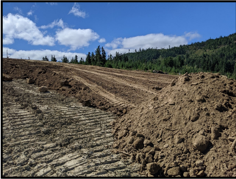
Picture # 5: Bulked in topsoil placed on the north side of the PEA prior to grading and track-packing.
