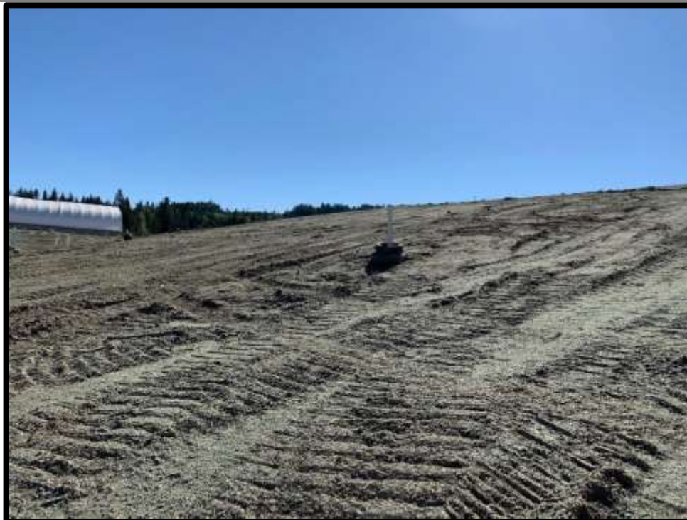
Picture # 4: Looking southeast, the PEA has been smoothed out and hydroseeding completed. Tires can be seen protecting the cleanouts and monitoring wells.
