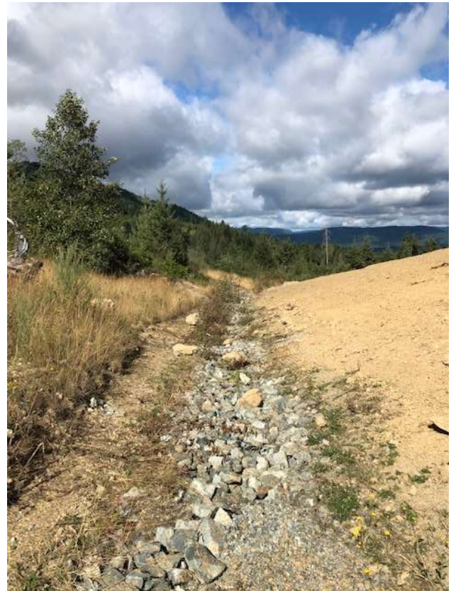
Picture #1 (left) : South ditch with more rip rap added to cover all geotextile
