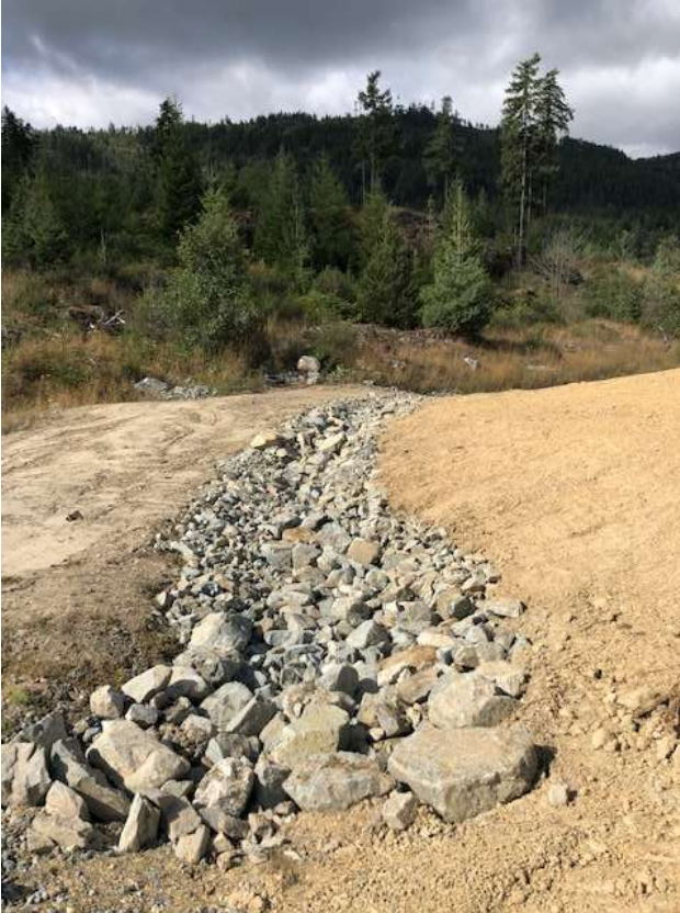
Picture #1 (left) : South ditch with more rip rap added to cover all geotextile
