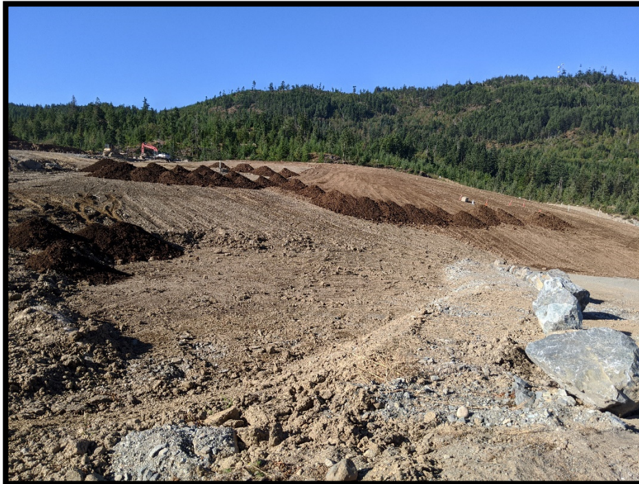
Picture # 1: Looking towards PEA from quarry entrance road – Contractor is moving previously stockpiled topsoil onto the PEA to increase thickness of cap, improve drainage and build out 5:1 slope.
