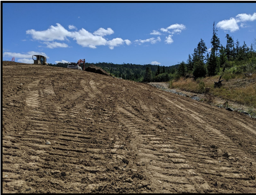
Picture # 6: Placed, graded and track-packed topsoil along the west side of the PEA. View is to the south.
