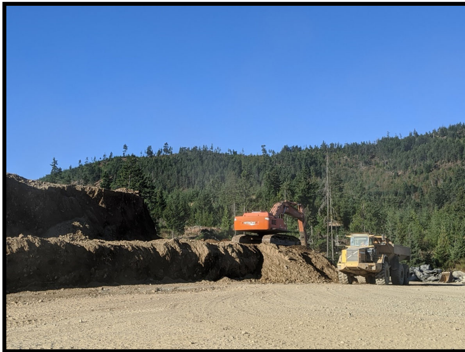
Picture # 2: Previously stockpiled topsoil material being loaded on to a rock truck. Larger rocks or unsuitable debris were removed from the topsoil prior to being loaded on to the rock trucks.
