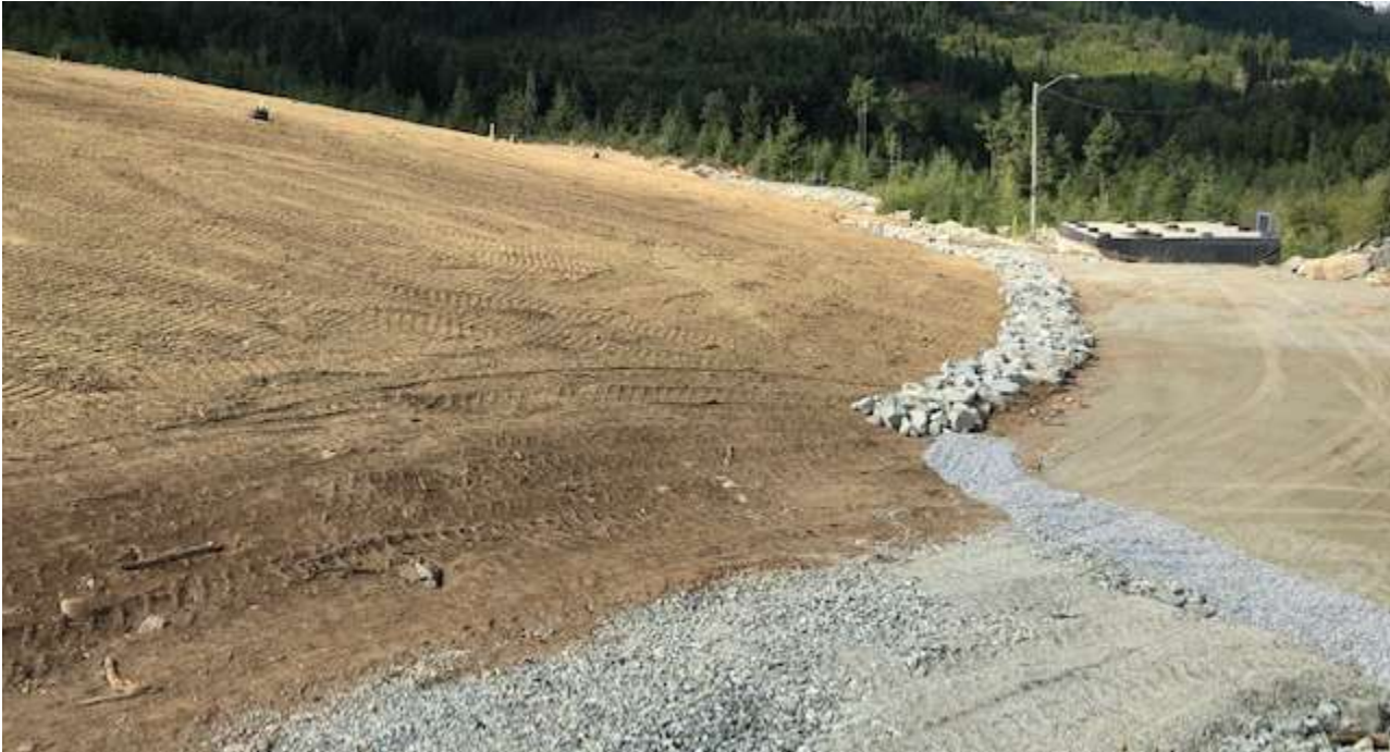
Picture #6: North slope toe extended to achieve 5H:1V slope.
