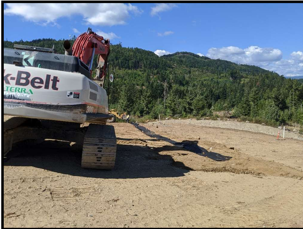
Picture # 4: Looking west along the north slope of the PEA towards the contractor installing a drainage control ditch. Geofabric was placed along the ditch prior to placing clear crush material. Drainage ditches are expected to be completed by tomorrow.
