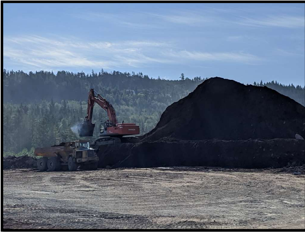
Picture # 3: Stockpiled topsoil material being loaded onto a rock truck to on-site transportation.
