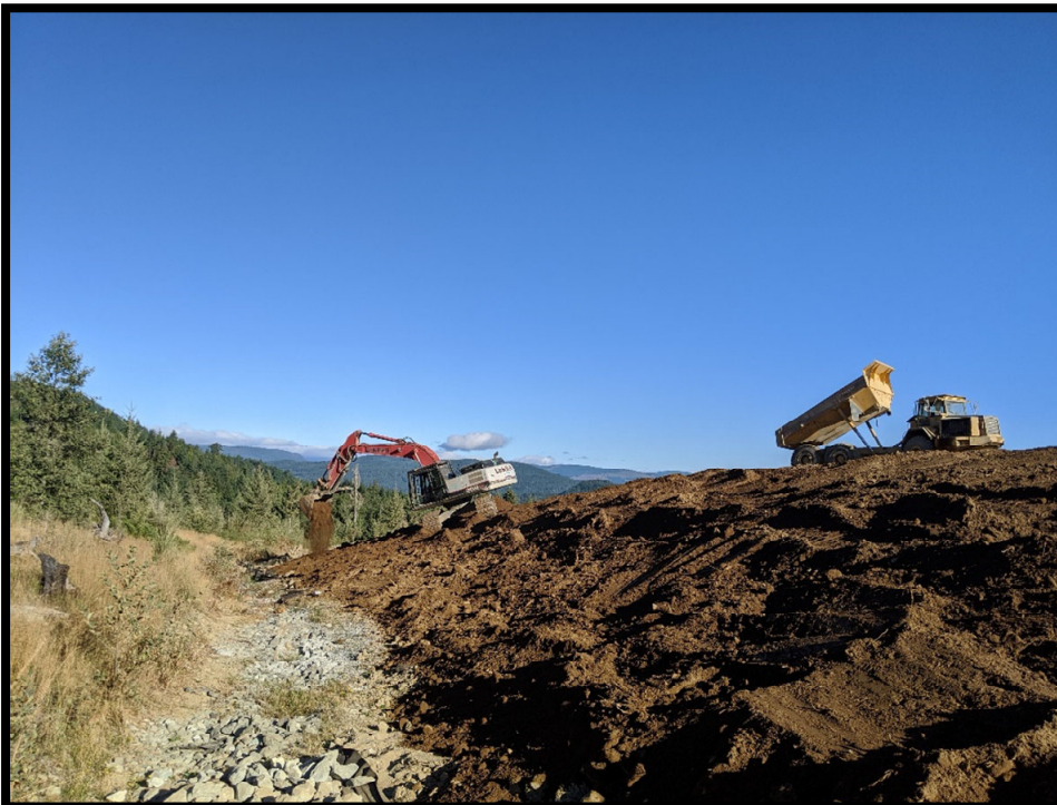
Picture # 4: Looking north along the western slope of the PEA towards topsoil being placed and graded.
