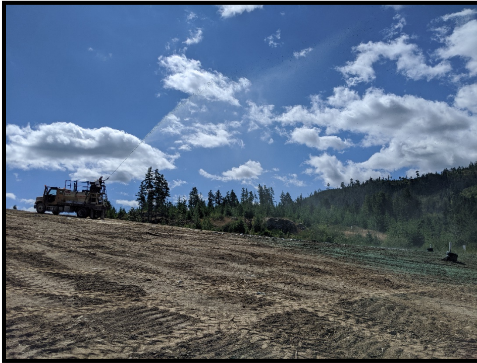
Picture # 1: Hydroseed contractor was on site for the duration of the day hydroseeding the previously placed topsoil over the PEA. View is to the southwest.
