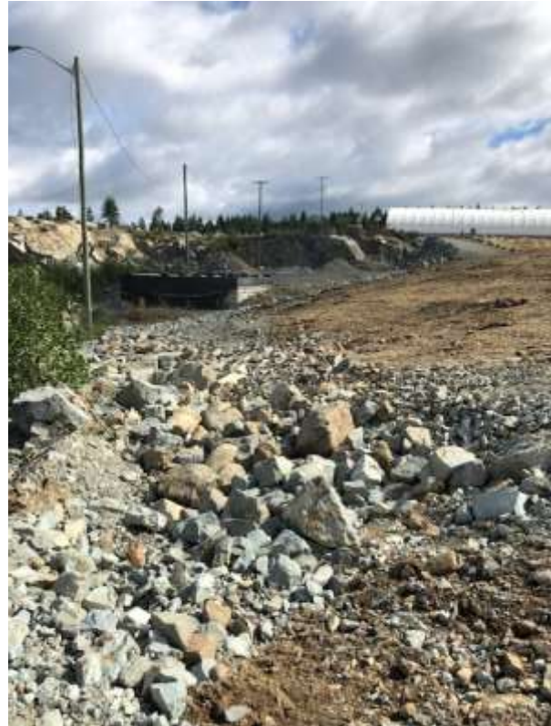
Picture #4 (right): Berms knocked down and sloped to match cover
