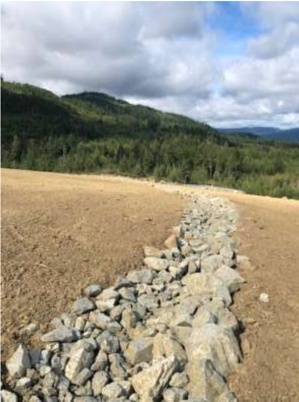
Picture #3 (left): Intermediate ditch complete
