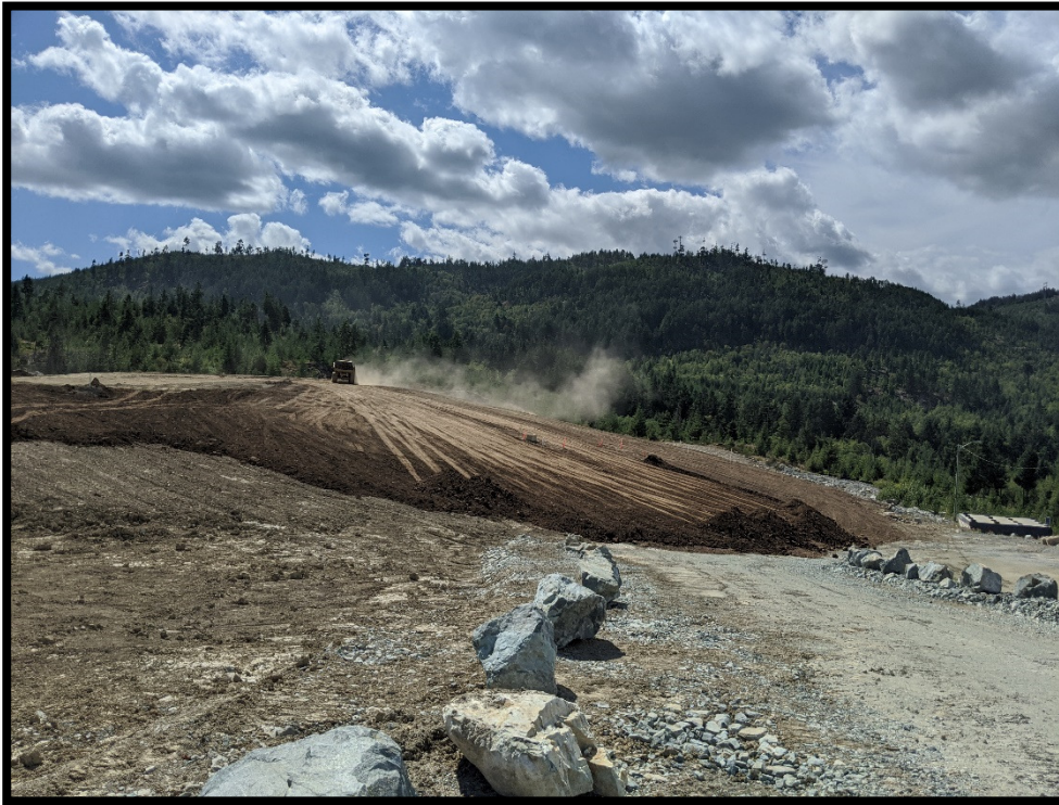
Picture # 3: View of PEA from quarry entrance road. Materials dumped onto PEA earlier in the day have been spread with dozer.
