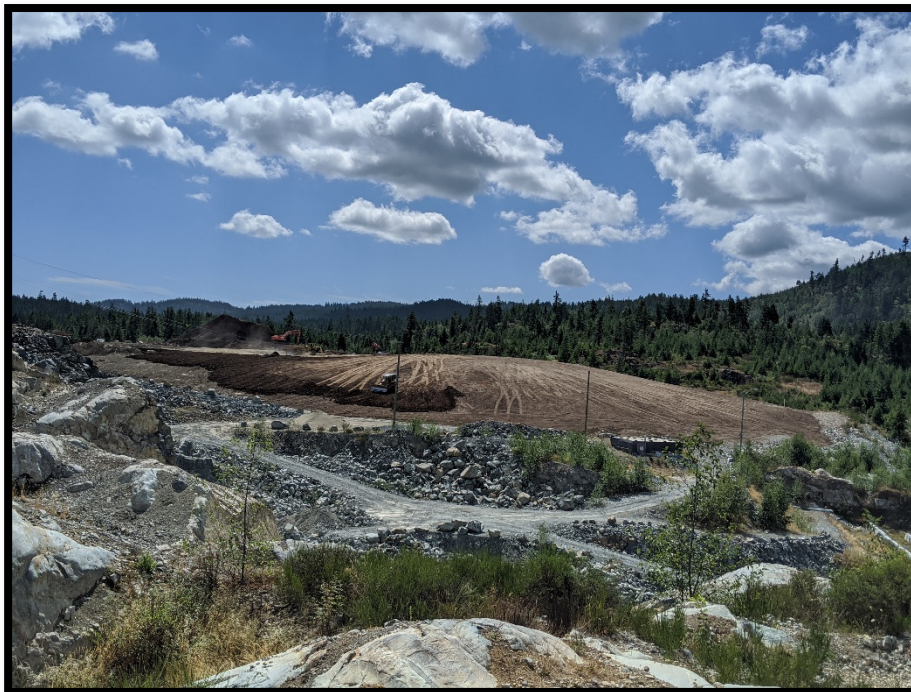
Picture # 2: Overview of PEA, looking south. Dozer is spreading soils down PEA slope.
