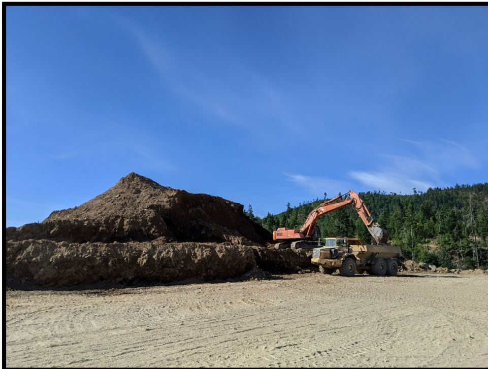
Picture # 2: Previously stockpiled topsoil material being loaded on to a rock truck for transport.
