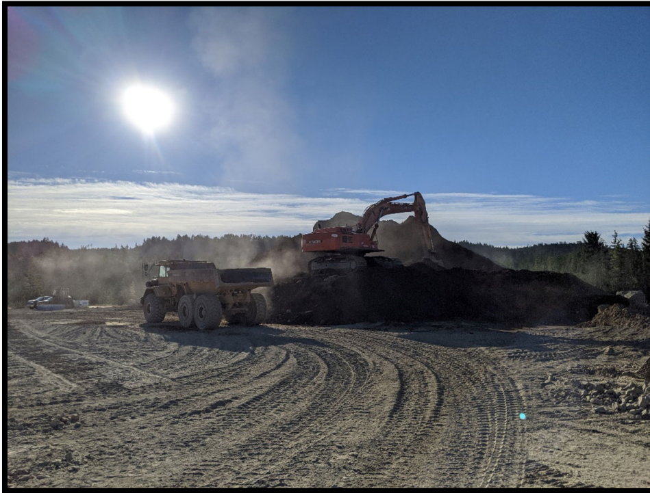
Picture # 3: Looking southeast towards an excavator loading a rock truck with stockpiled top soil material.
