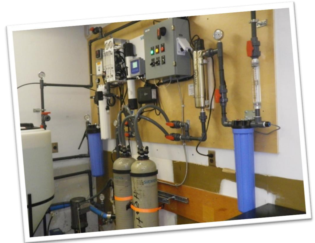
Reverse osmosis and demineralization system in situ
