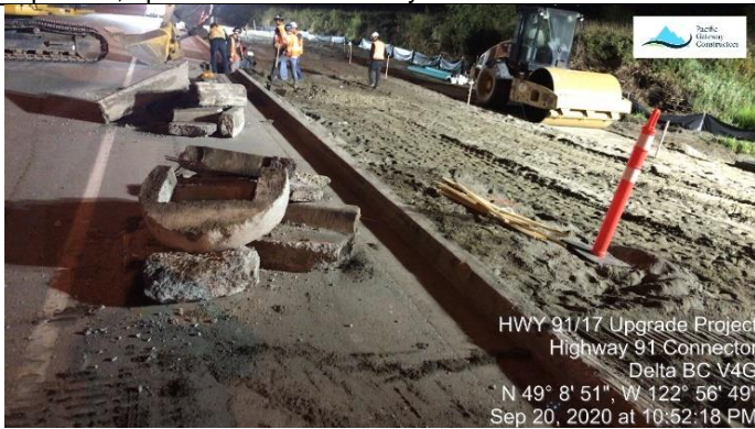
Photo 9. Catch basins removed in preparation for the installation of new ones at C01 Detour.
