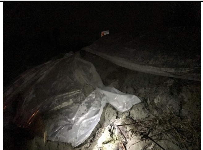
Photo 24. Poly sheeting covering exposed sand stockpiles at 96 Street Ditch.
