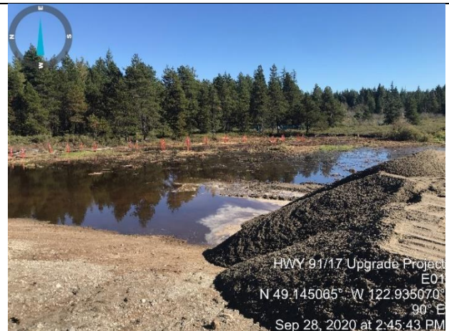
Photo 26. Stockpiling of sand at the Delta Nature Reserve for the preload.
