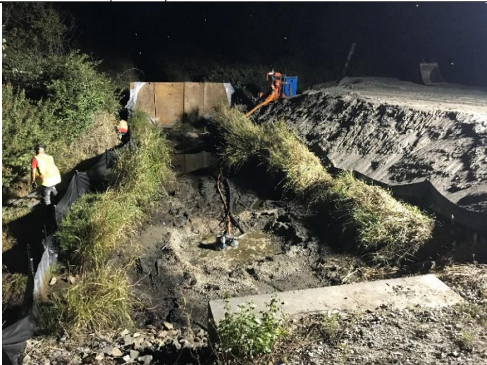
Photo 5. 96 Street Ditch (area B) isolation for the culvert extension.
