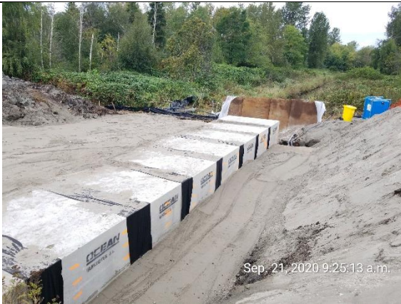
Photo 7. 96 Street Ditch culvert extension installation and compaction, upstream view from Hwy 17.
