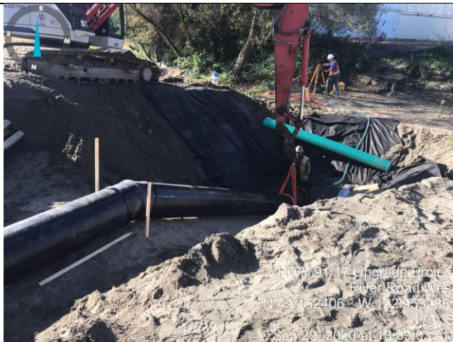
Photo 25. River Road west (Site C), continuing watermain installations.
