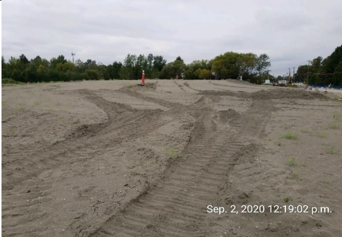
Photo 1. Most working surfaces had been covered with sand preload such as River Road west (Area C).
