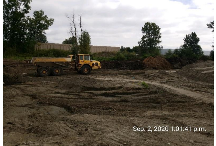
Photo 2. Topsoil stripping was underway at River Road east (Area D). Erodeable soils were contained within a basin.
