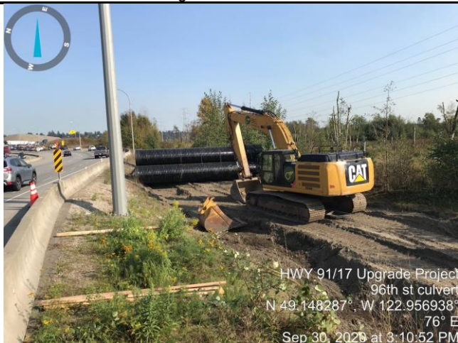
Photo 23. Delivery of culvert sections on the south side of the 96 Street Ditch.
