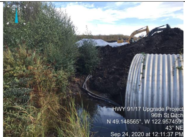
Photo 14. 96th Street Ditch culvert extension, poly covering stockpiles, view to the east.
