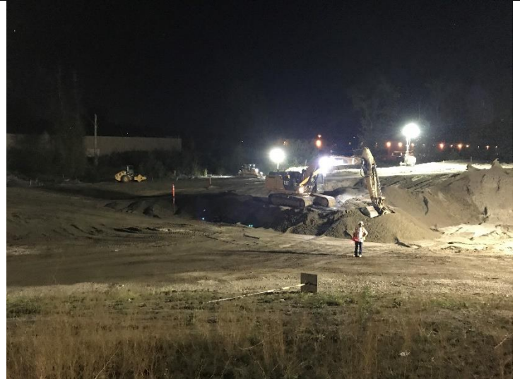
Photo 4. Most working surfaces had been covered with sand preload River Road West. Erodeable soils were contained within a basin.
