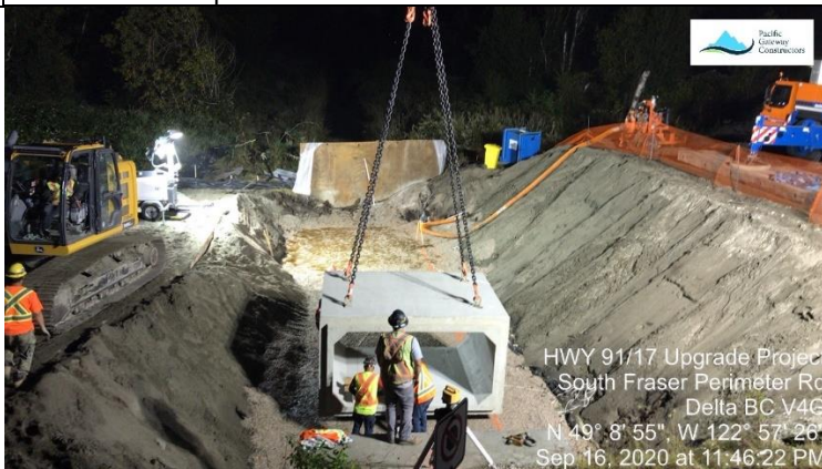
Photo 15. Placement of culvert section in the 96 Street ditch channel, upstream view from Hwy 17.
