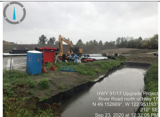
Photo 12. Heavy rainfall caused River Road ditch water level to rise and swamp ECS fence but still intact.
