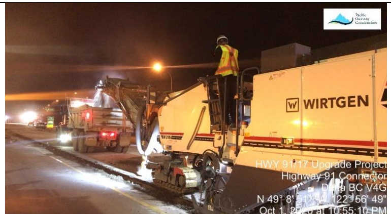
Photo 28. C01 removal of the existing medium by way of milling.
