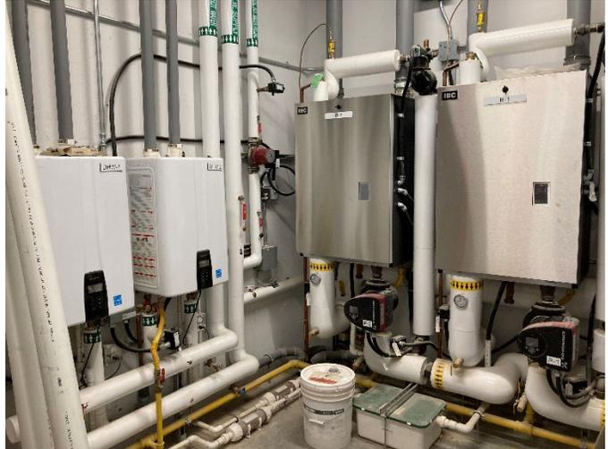
*New high efficiency, on-demand hot water heating (L) and boilers (R) at wə́kʷaṅəs tə syaɣʷəm Elementary School*
