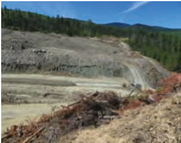
Backfill going over Pole Cutters Creek box culvert
