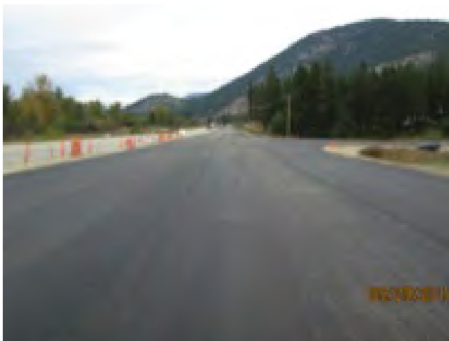
Bottom lift paving of L100 EB lanes
