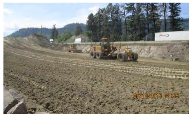
Placing Type 'D' fill at 131+00 to 132+60
