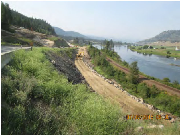
Type 'D' embankment at 140+00 - 142+00 c/w rock blanket.
