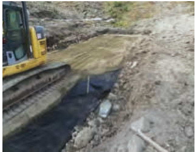
Sunday Creek North Fork box culvert foundation bedding placement
