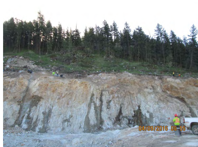
Installation of mesh anchor and cable system – East rock cut
