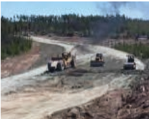
Type D/unsuitable materials placement and compaction
