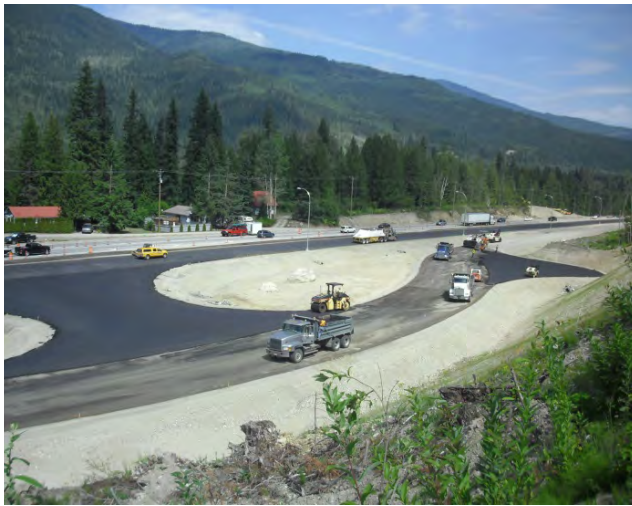
Bottom lift paving on L100 (Highway 1) and L400
