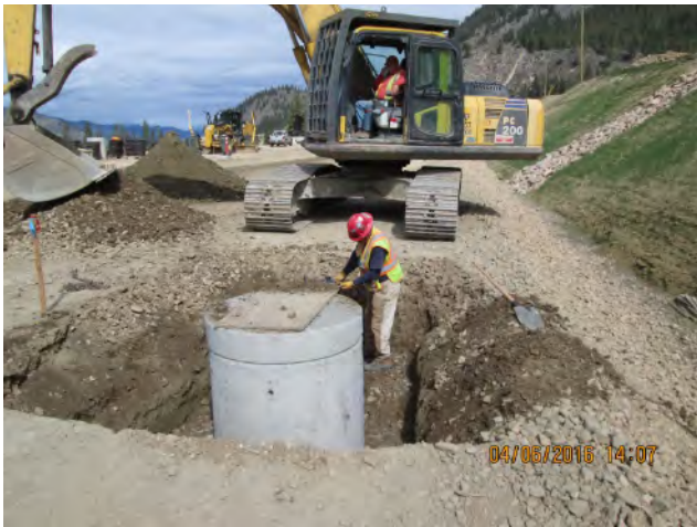
Installing CB barrels 126 - 131
