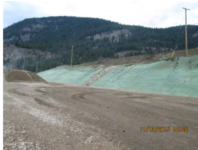
Hydroseeding West cut slopes
