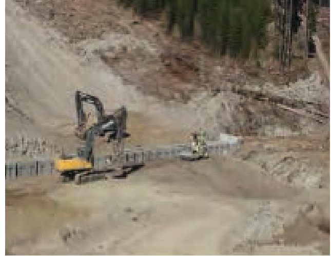
Sunday Creek South Fork box culvert backfill
