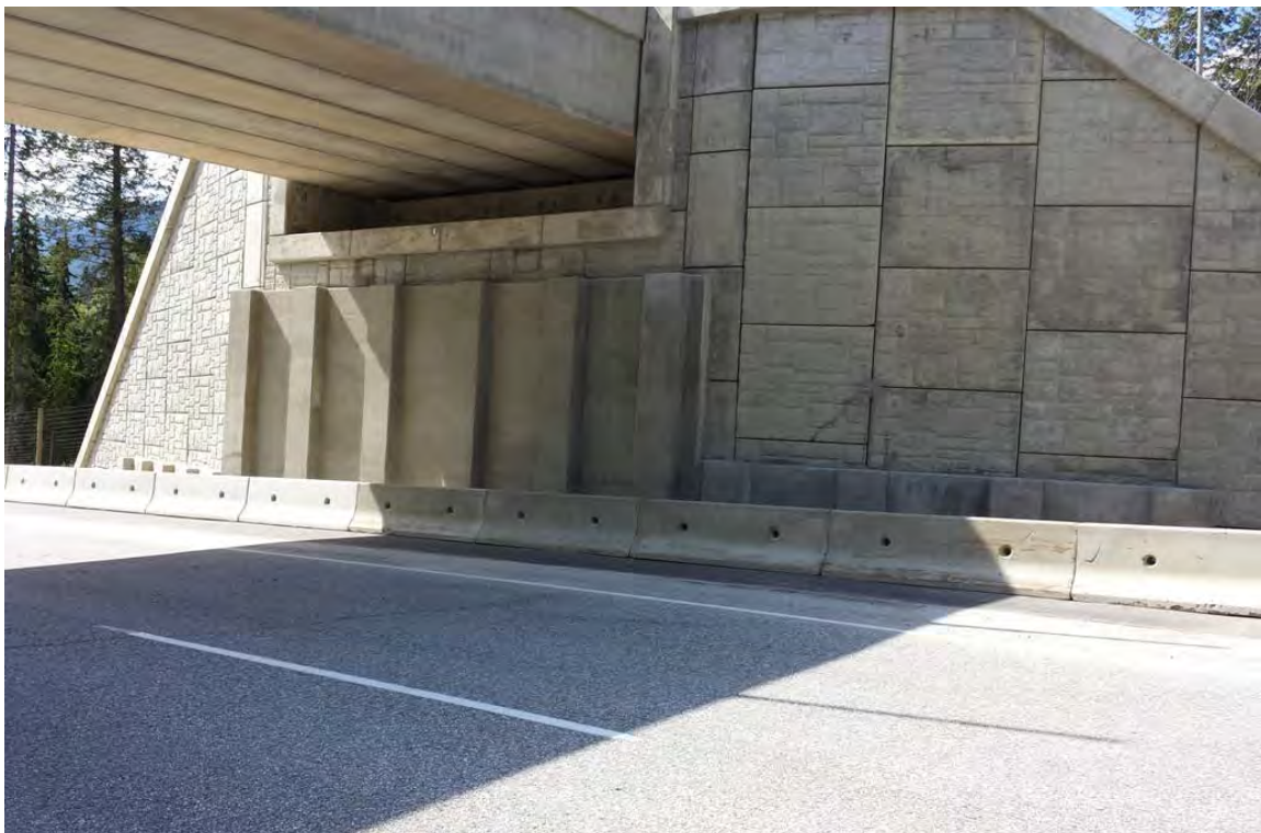
MSE Wall Repair Complete 2014
