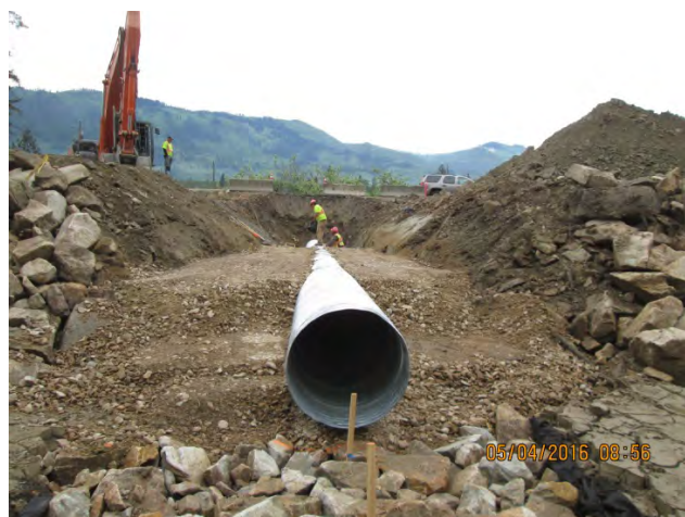
1,000 mm CSP install at 131+60
