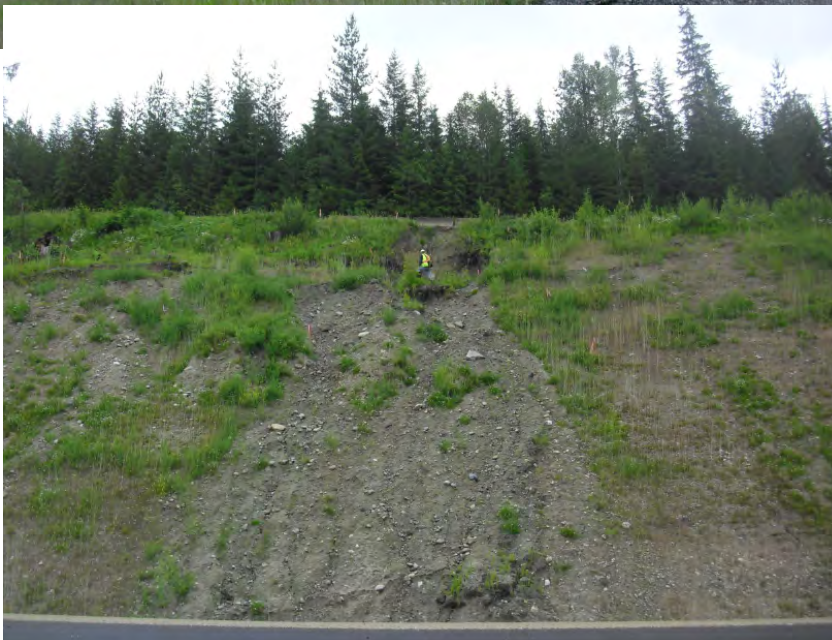
A slope failure above the L 400 Line and on the shoulder of Sederburg Road will require additional work to the contract which will involve a rock buttress wall and rock fill to stabilize the slope. This work to begin on June 17, 2016 and is anticipated to take 10 to 12 days.
