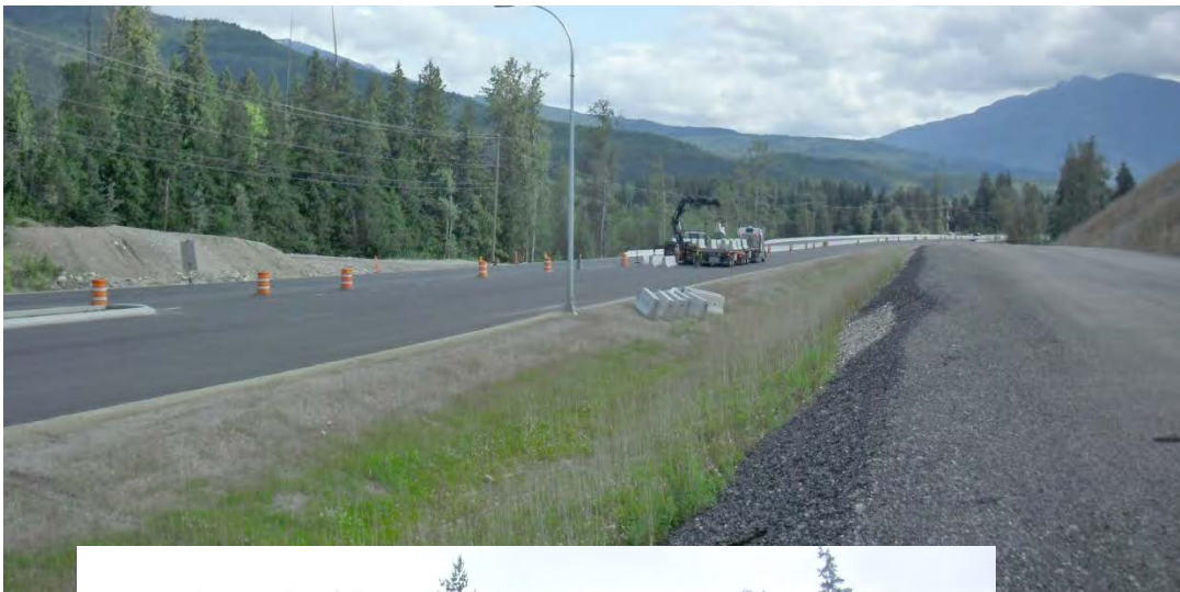
Concrete median barriers being placed
