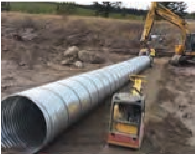
900 mm CSP installation
