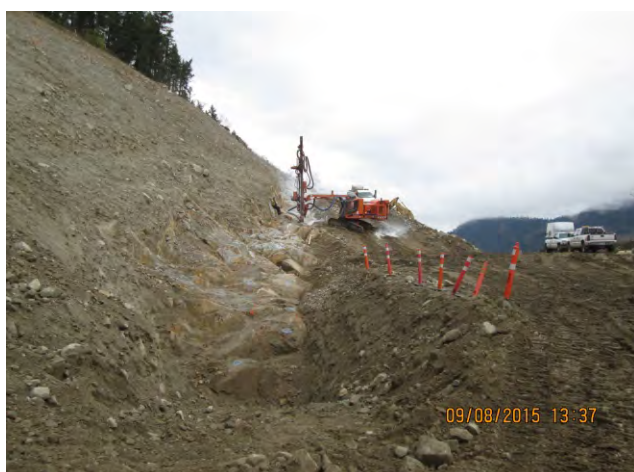
Drilling for Wall #4 Dewy Dag Anchors
