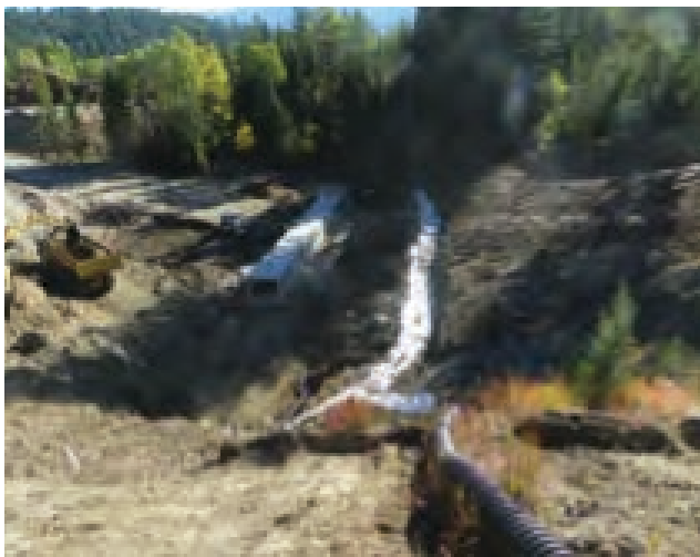
Sunday Creek North Fork box culvert install and water diversion
