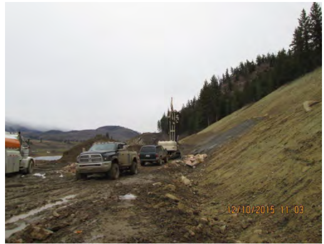
Geotechnical core drilling at 139+40 blue clay area
