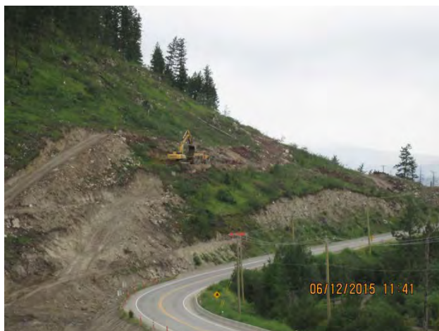
Type 'D' excavation for Wall #4
