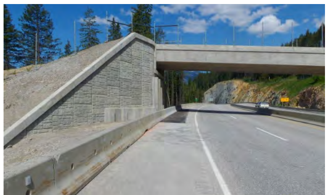
MSE Wall Repair Complete – Glenogle 19 June 2014
