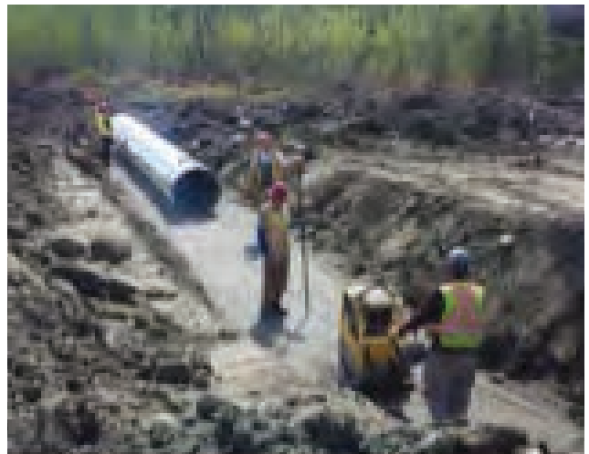
Culvert installation
