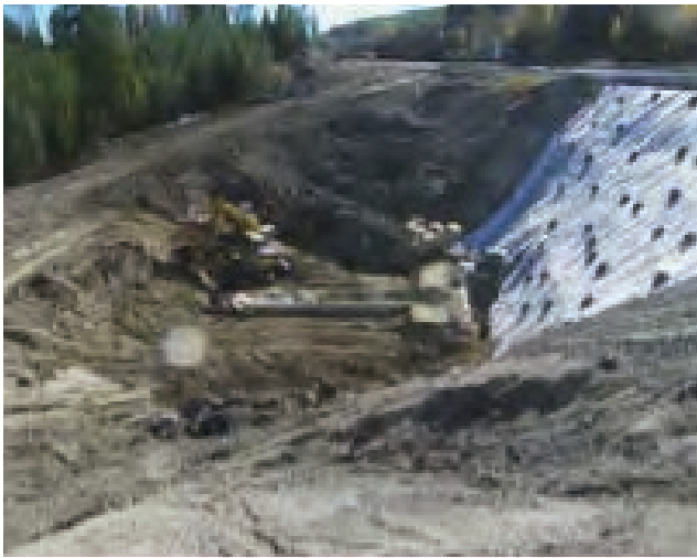
Sunday Creek North Fork box culvert install and backfill
