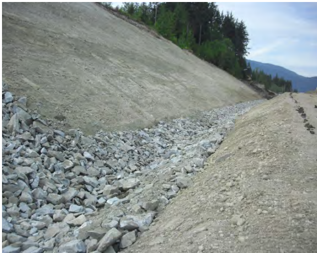
Rip Rap ditch, south side of L400 Line
