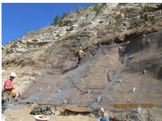
Teco mesh installation at 132+55 – 133+10
