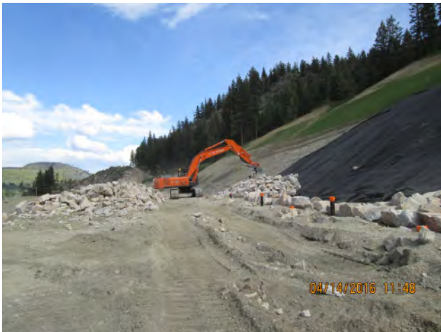
Rock buttress construction 139+25 – 139+55
