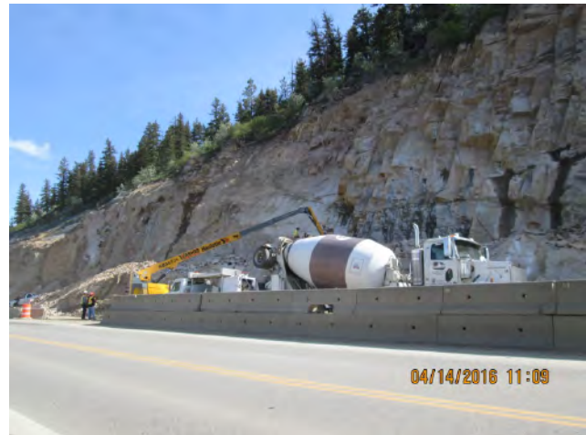
Prepping for shotcrete at overhang repairs 134+15
