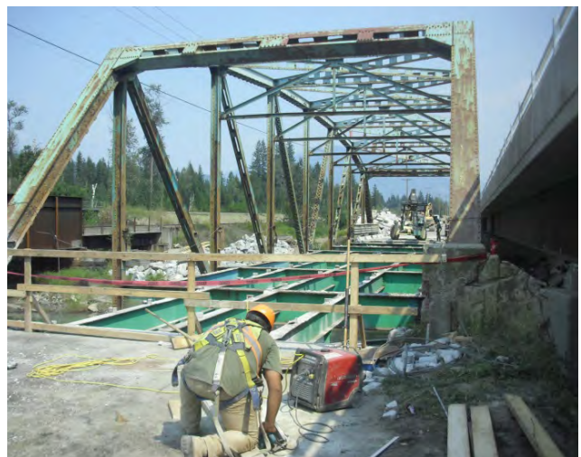
Existing bridge demolition works
