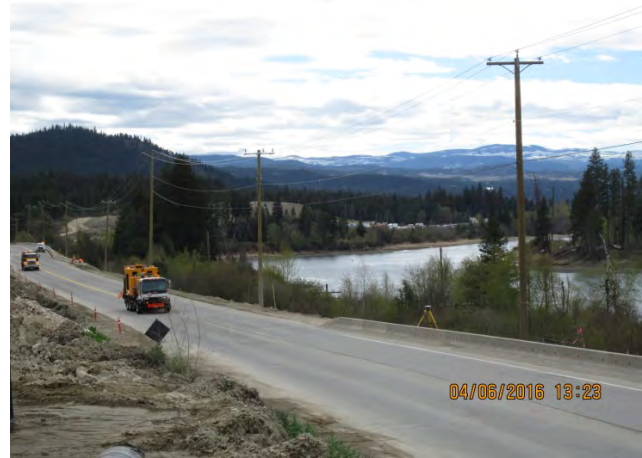
Repainting centerline through detour #1 and #2
