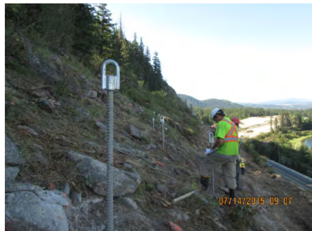
Mesh anchors installed
