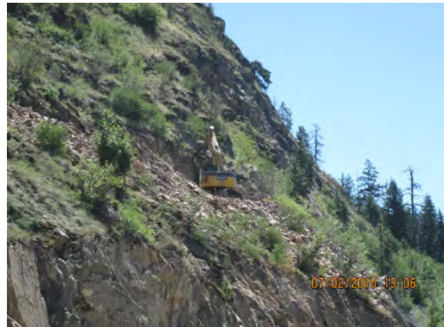
Rock hammering pioneer trail at 133+80
