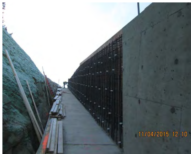
Wall #4 rebar and forms
