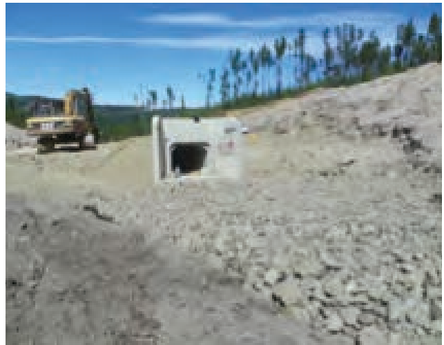
Pole Cutters Creek box culvert inlet structure and rip rap protection
