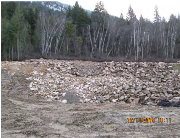
Blue Clay buttress drain at 138+00 constructed to elevation 365.60 m
