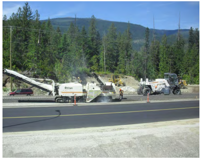
Pulverizing existing Highway 1
