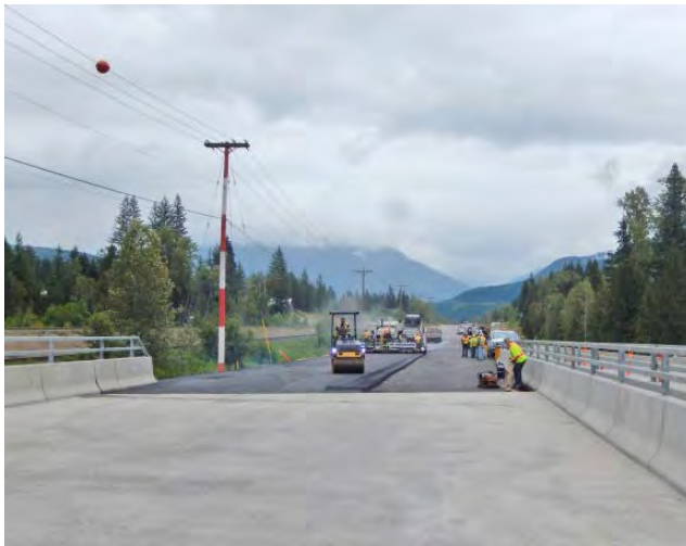
Paving top lift from the completed Westbound bridge
