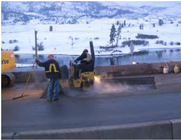
Paving patch repair at 141 Westbound
