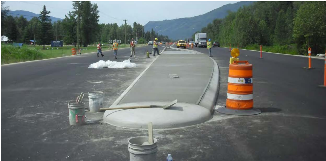
Concrete infill of median curb
