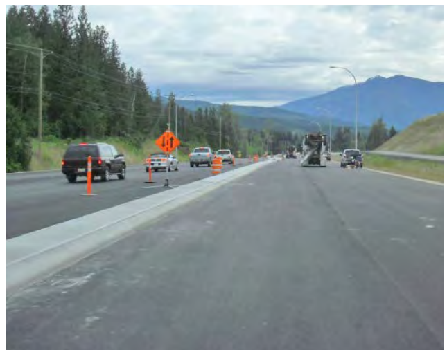
Concrete medians being placed on top lift pavement. Completed June 16, 2106
