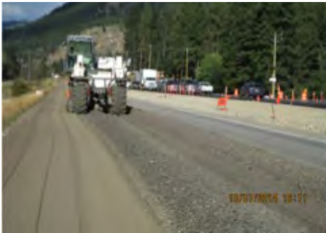
Pulverized old existing WB lanes from 110+00 to East LOC 127+30
