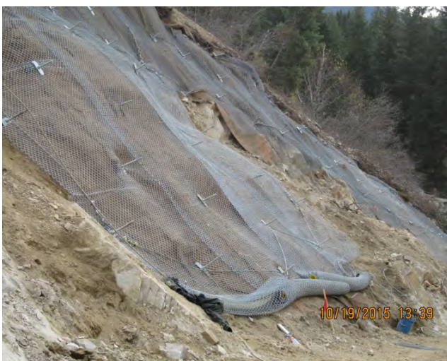
Extra "Teco Mesh" required at 132+90
