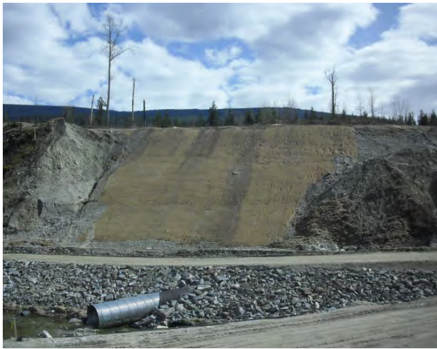
Coco matting placed on L400 Line slopes
