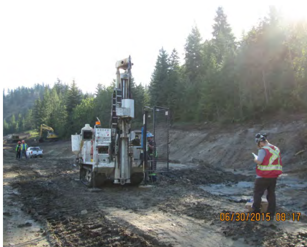
Drill rig at 138+00 to investigate blue clay
