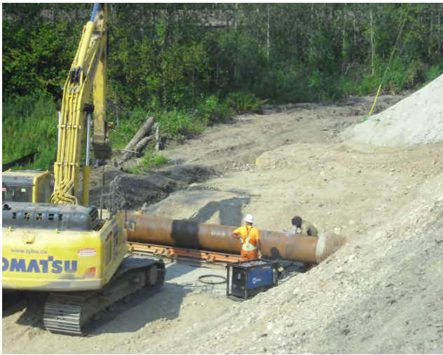
SA #2 works, welding and augering 750 dia. sleeve
