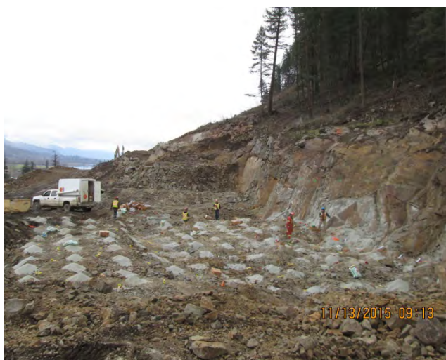
Loading blast at East rock cut 144+50
