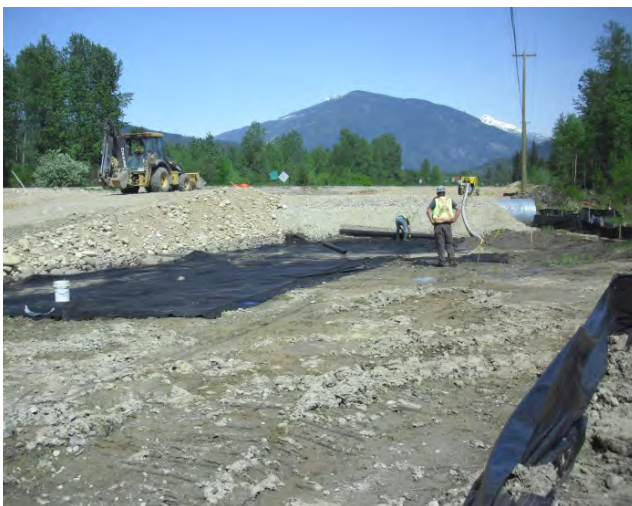
SA #1 works, placing geo grid and filter fabric
