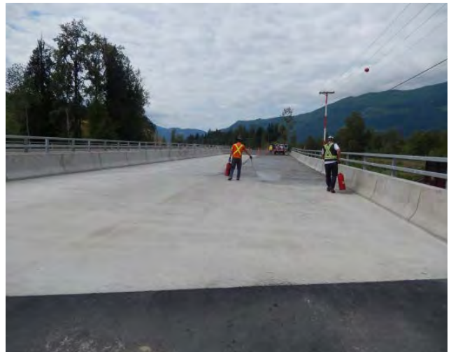
Linseed oil being applied to the new Westbound bridge which was constructed to replace the existing bridge
