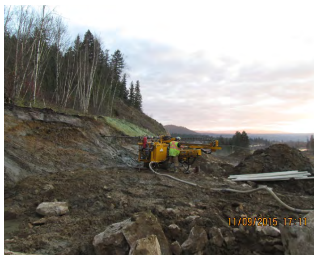
BAT Drilling dewatering pipes at 138+00 blue clay zone
