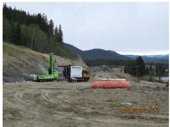
Drill depressurization wells at 139+25 – 139+55
