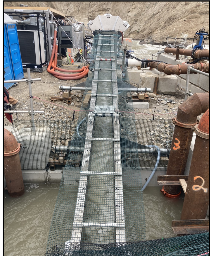
TOP: Mesh installation over the steep pass to prevent escape.
