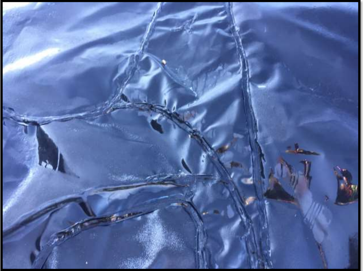
Photo 14 – Liner seams show no signs of deterioration
