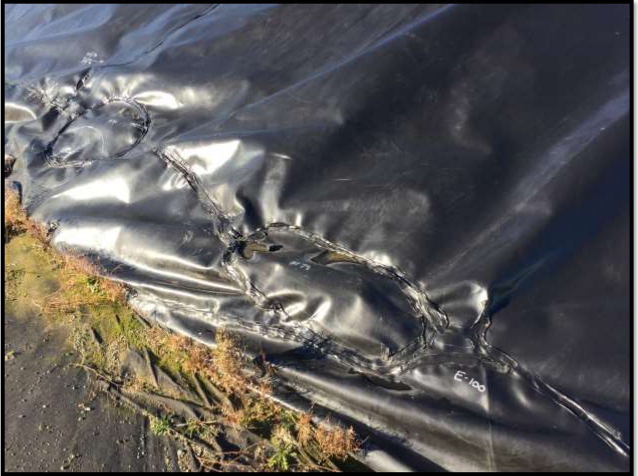
Photo 17 – Liner seams show no signs of deterioration
