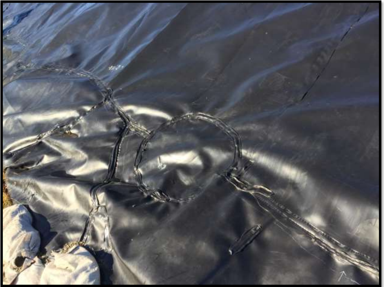
Photo 18 – Liner seams show no signs of deterioration
