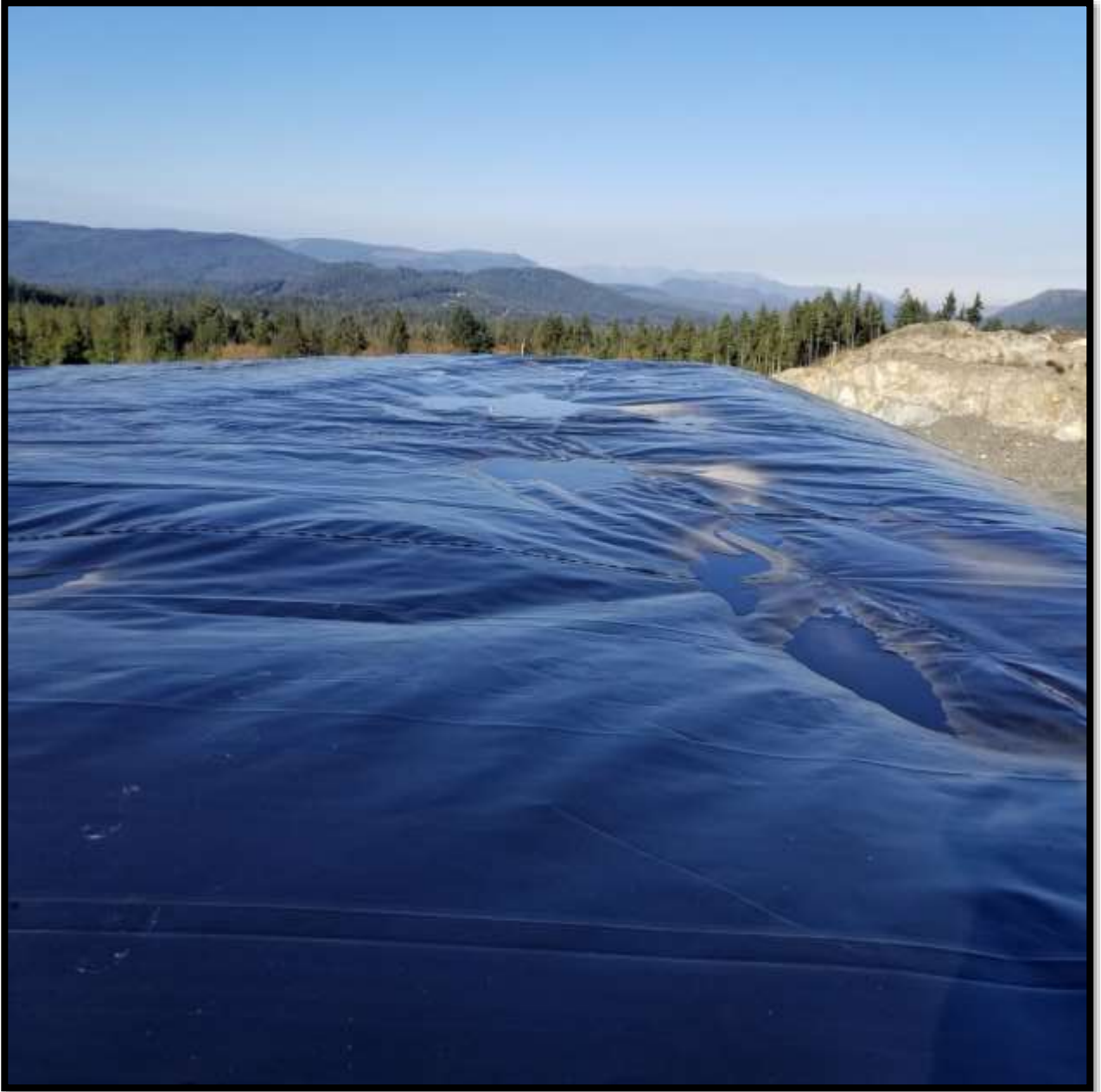
Photo 8 – Minimal ponding of surface waters is observed
