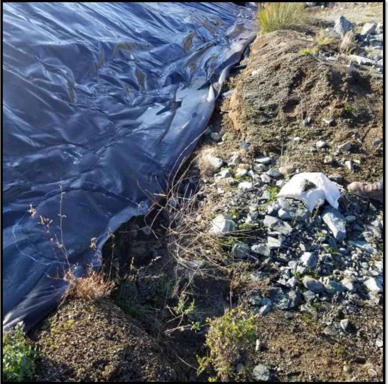
Photo 10 – Slight erosion of the quarry is noted at the NW toe-the liner is fully sealed at this location
