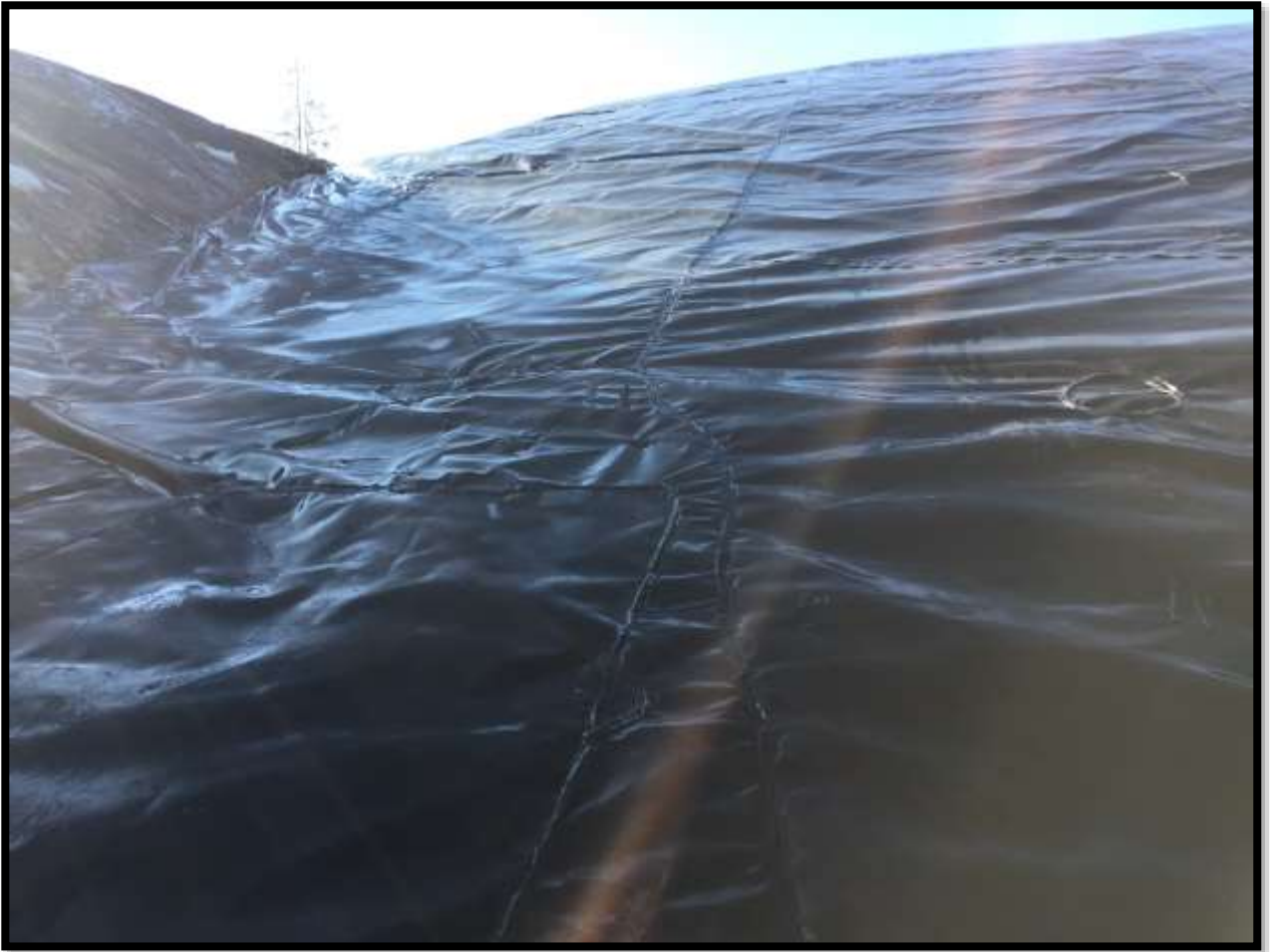
Photo 16 – Liner seams show no signs of deterioration
