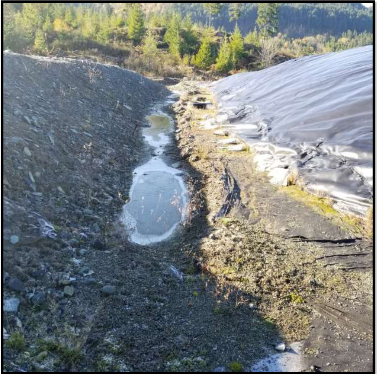
Photo 9 – South ditch erosion is not present
