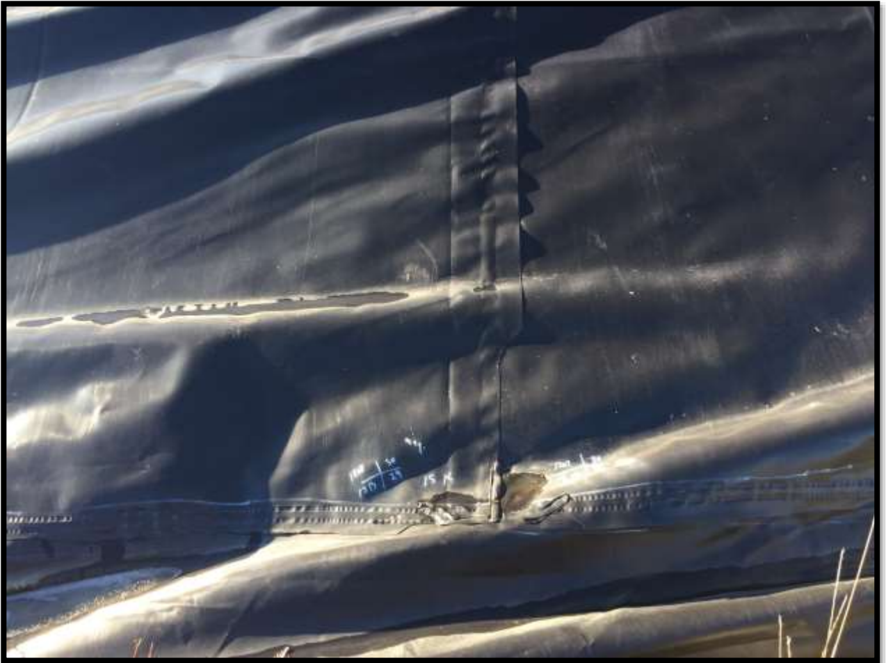
Photo 15 – Liner seams show no signs of deterioration
