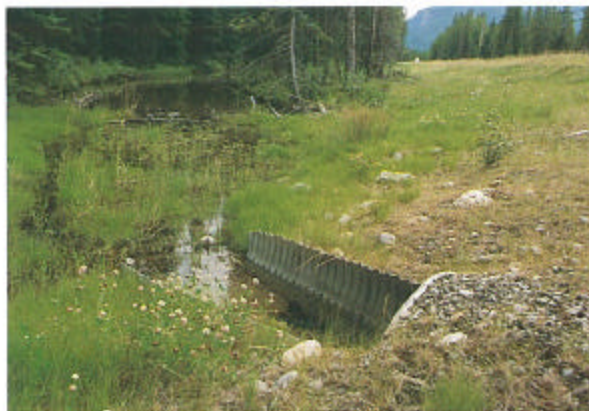
Figure A-4 This culvert outflow has been constructed to create an effective and well concealed transition between the pipe and stream.
