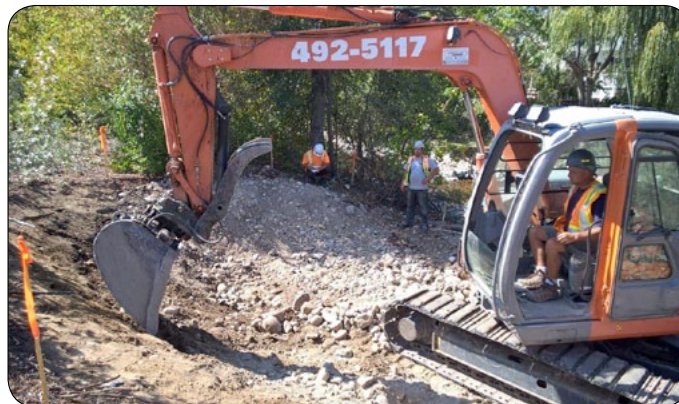
Constructing the bypass channel to help fish like kokanee and rainbow trout.
