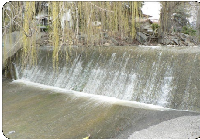
This concrete barrier prevented fish from travelling upstream.
