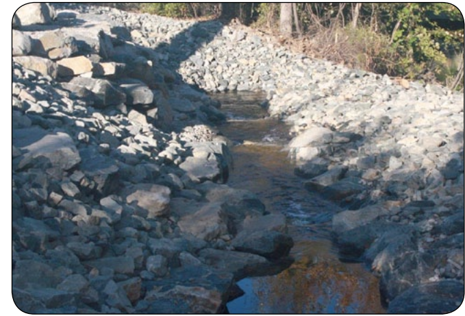
The bypass channel is a series of steps and pools.
