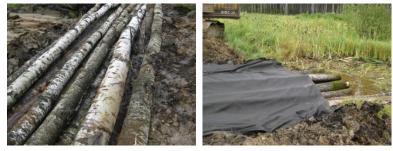
Example of a log bundle built 2 or more logs high with a separation layer placed over the top to prevent the voids from becoming filled with road surfacing material. The bundle was used to allow low volume flow through a road in a wetland. Note the logs extend past the edge of fill to allow water to easily enter or exit the structure.
