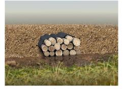
Exposed log bundle (left) made from a single row of logs needs complete reconstruction, and sediment control is required at the outlet. Log bundle built 2 or more logs high (middle) shows the open voids between boles and a straw bale at the outlet acting as a check structure to contain sediment.
