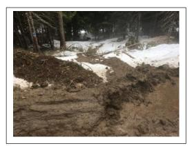
Exposed log bundle (left), ponded water (middle) and sedimentation (right) are examples of poor performance requiring mitigation; reconstruction, relocation, or choice of a different structure, such as a culvert, should all be considered.
