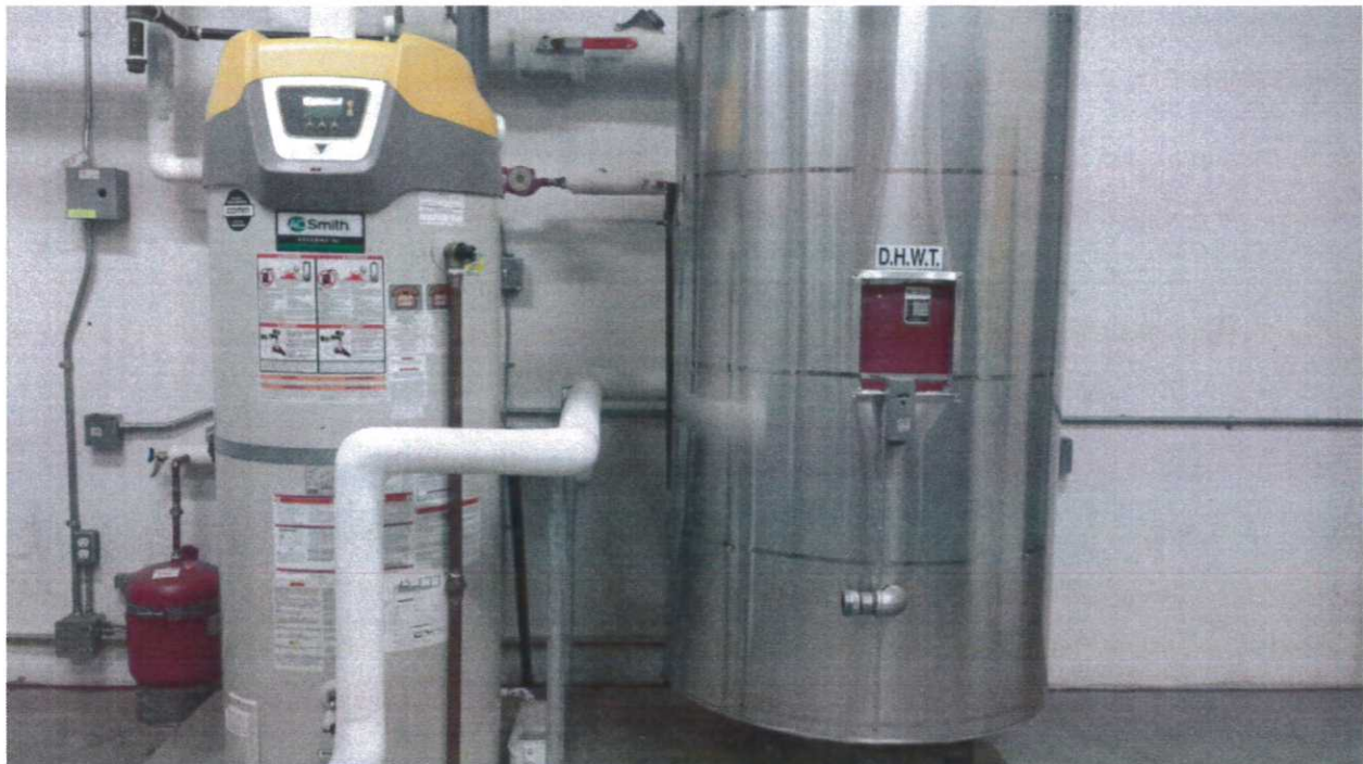
The new (AC Smith) and old domestic hot water tanks side by side at Queenesh Elementary
