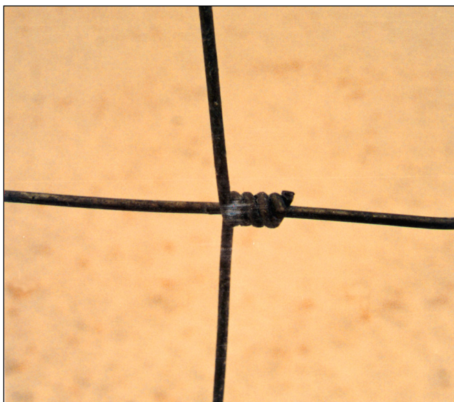
Figure 2 Hinged Joint
