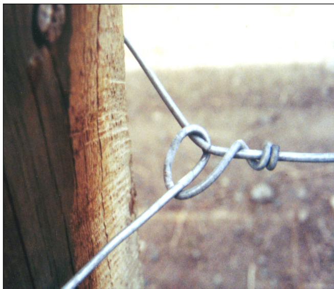
Figure 6 Tying Off Woven Wire (top view)
