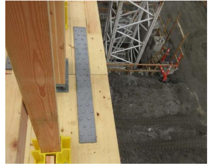
Steel drag-straps
