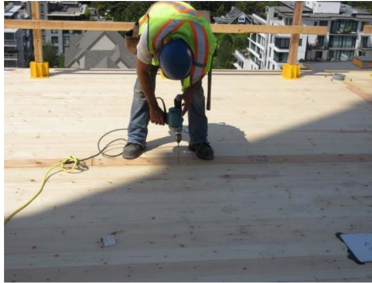
Plywood splines
