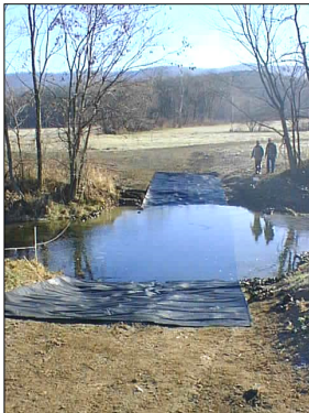
Geotextile Laid
