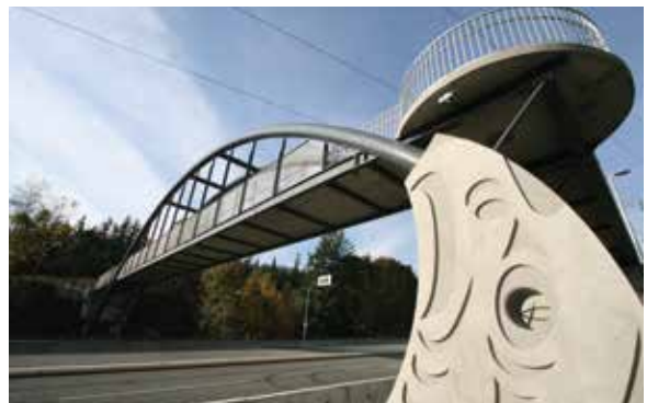
Highway 99 Squamish Pedestrian Overpass
