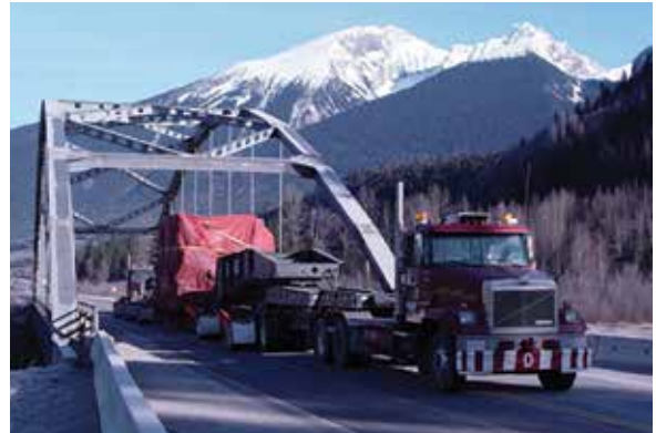
Upper North Thompson Bridge – Highway 5
