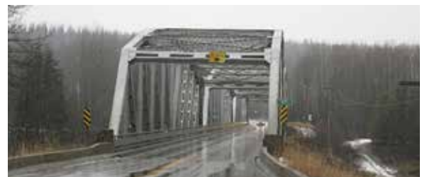
Parsnip Bridge, Highway 97
