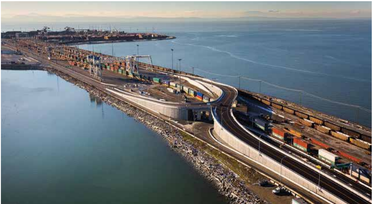
A new overpass on Roberts Bank causeway, separating road and rail traffic, opened in October 2014
