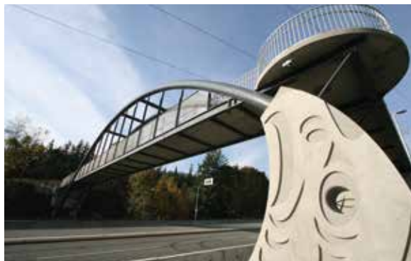
Highway 99 Squamish Pedestrian Overpass
