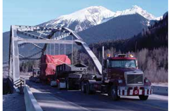
Upper North Thompson Bridge – Highway 5
