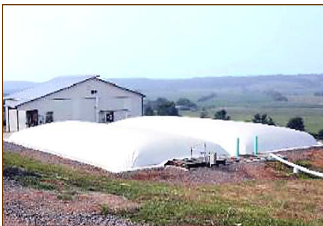
Figure 1 A medium-scale on-farm “covered lagoon” biogas facility for manure on a US dairy farm.
