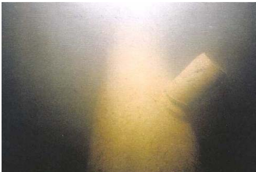
Figure 7: Outfall inspection of diffuser port.
