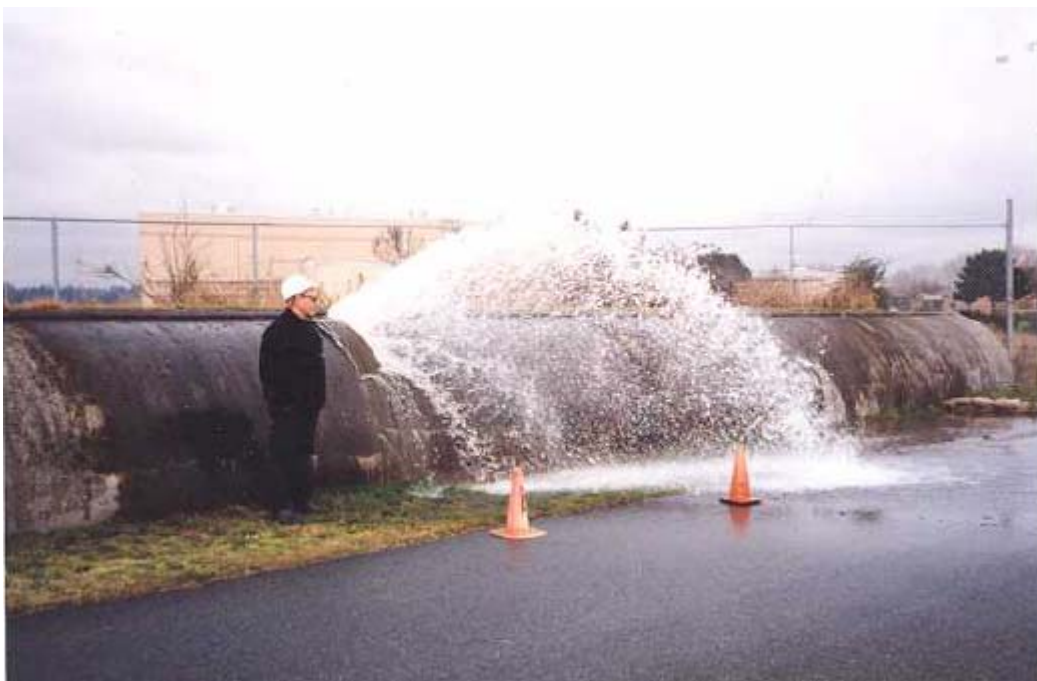
Figure 8: Leak from an effluent outfall conduit at a large wastewater treatment plant (courtesy GVRD).
