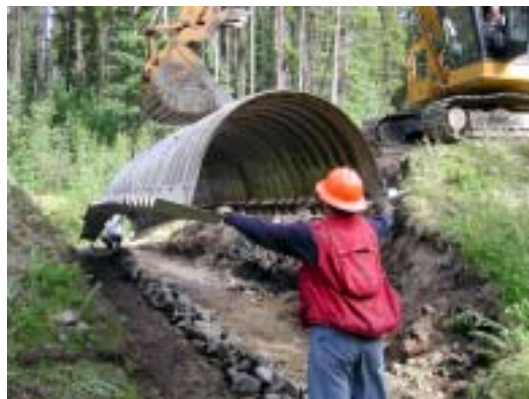
Figure 11. Excavator and workers orienting arch for final placement.
