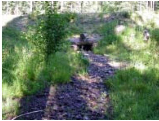
Figure 2. Inlet of Barton Road wooden-box culvert.
