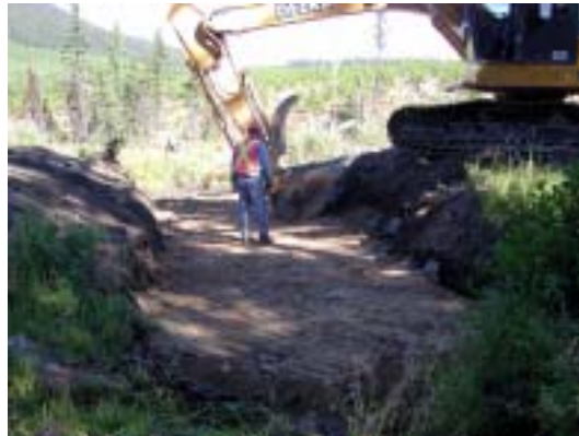
Figure 9. Compacting the final lift with the excavator bucket.
