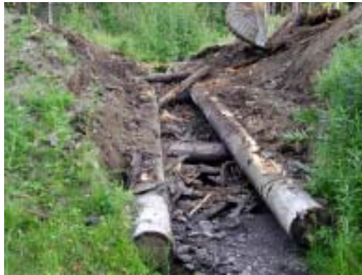
Figure 6. Excavator removing final stringers from over the sill logs.
