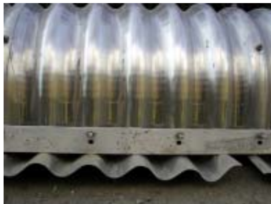
Figure 5. Corrugated aluminum arch and footings showing the corrugation profile and gap between the footing sections.
