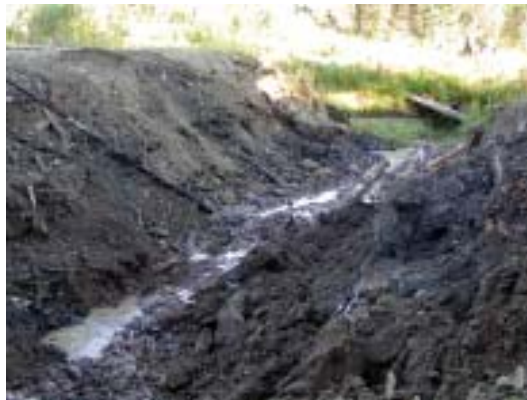
Figure 7. Excavated trench at Esperon Road site.
