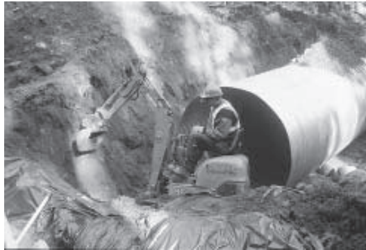
Figure 7. A Kubota K008 mini-excavator spreads material within the CSP.
