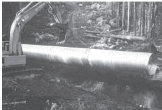
Figure 5. The excavator placed the CSP into the excavated trench.
