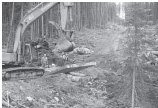
Figure 3. Temporary structure being dismantled.
