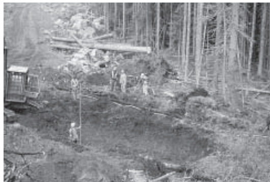
Figure 4. A surveyor and helper took measurements within the excavated trench.
