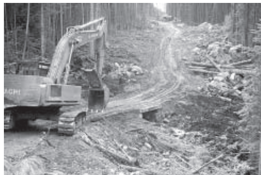
Figure 1. View of stream crossing, showing newly built road and temporary structure.
