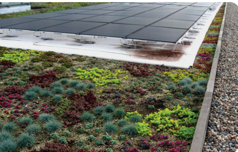
The new Port Coquitlam Driver Licensing Centre features a green roof to cool the building and slow storm water run-off, as well as solar photovoltaic panels.
