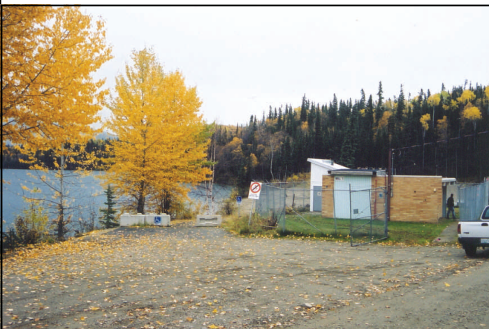
Plate 1. A view of the Mackenzie pump house where the raw water samples were collected. Morfee Lake is in the background.
