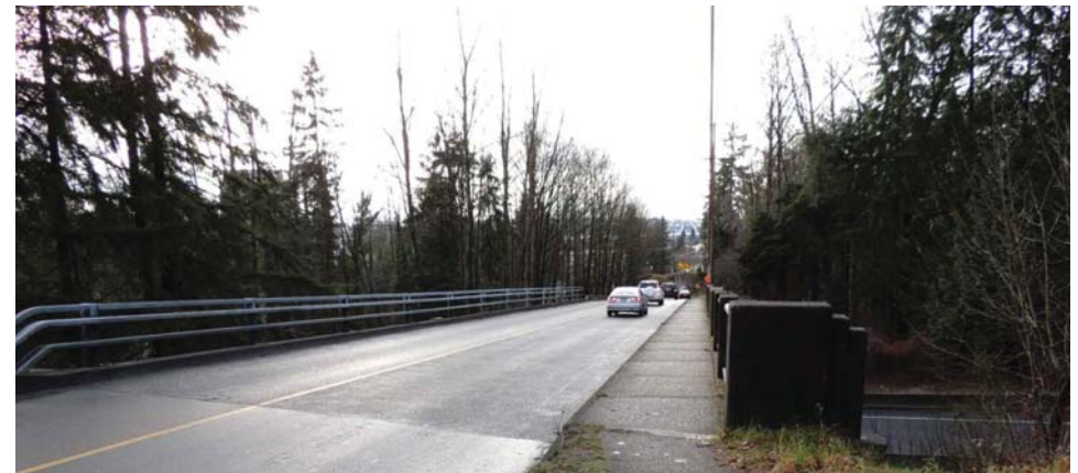
Mountain Highway Overpass – looking south towards Keith Road
