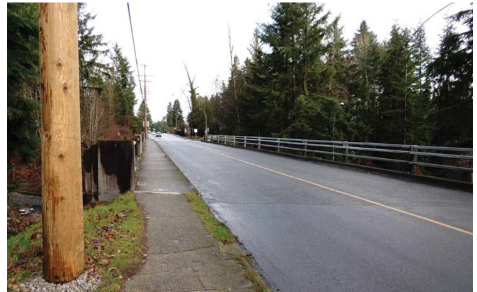
Mountain Highway Overpass – looking north towards Arborlynn Drive
