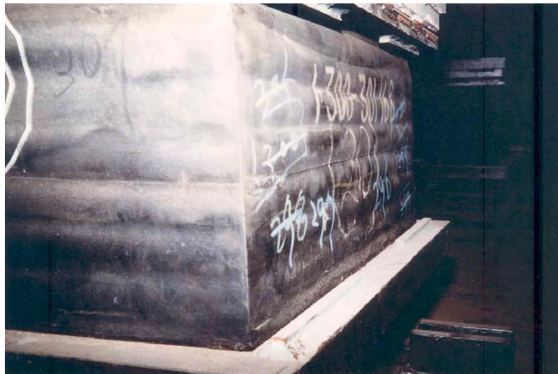
Figure C11.6.6.8.f.4 Evidence from the bulges that the top plate is bent along the right face
