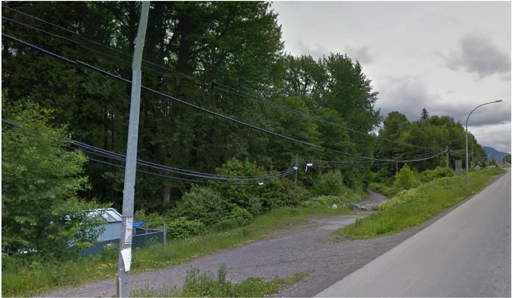
Looking south along Lakelse Avenue at the Thornhill Frontage Road – Note the overhead lines and public barricade as well as the utility building.
