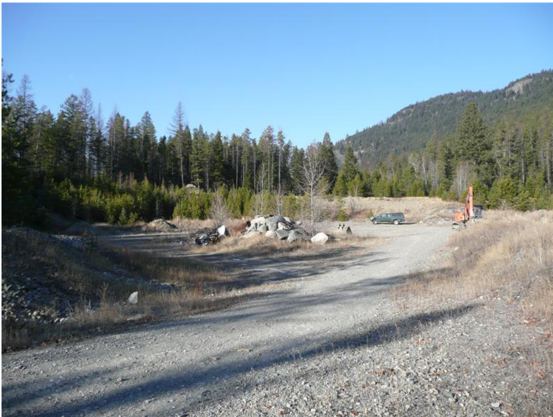
View of excavated pit area, potential crusher site location.
